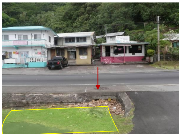
13B. A rain garden is proposed in the parking lot. Outlet into existing drain inlet is shown with the red arrow.
