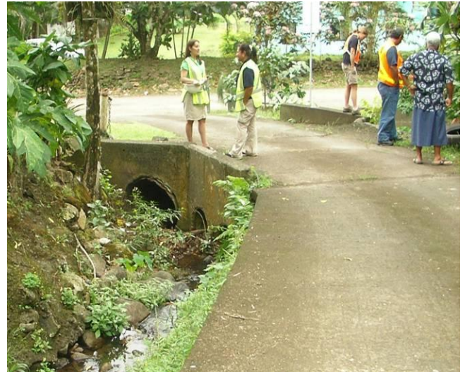
Figure 3A. Looking downstream towards the upper end of the three-pipe culvert.
