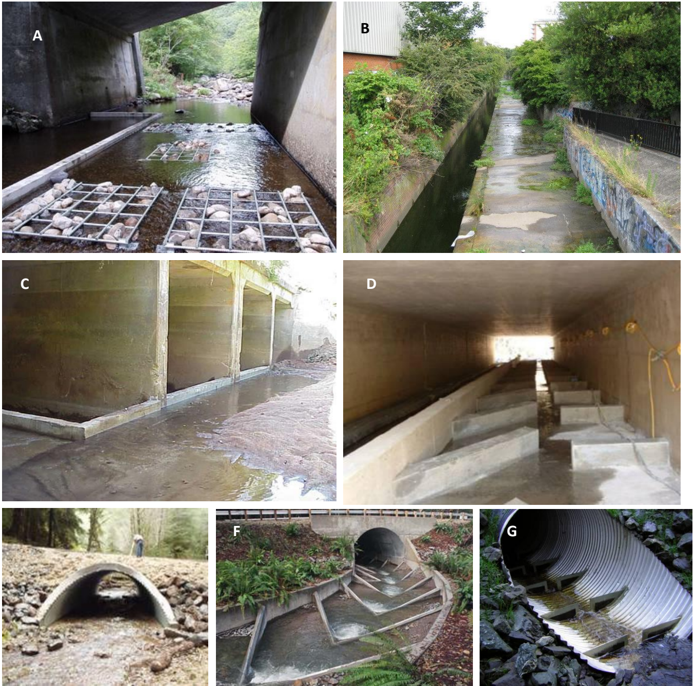
Figure 1C. Photos of various alternatives to create low flow channels using separator walls (A, C, D) coupled with baffle devices (A,D,F, and G); low flow channel within a larger high flow channel (B); and using open bottom/arched culverts to allow for natural bottom habitat.
