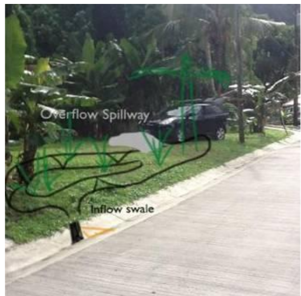
Figure 2A. Potential location for community bioretention to capture and treat a portion of the runoff conveyed in existing concrete roadside swale.
