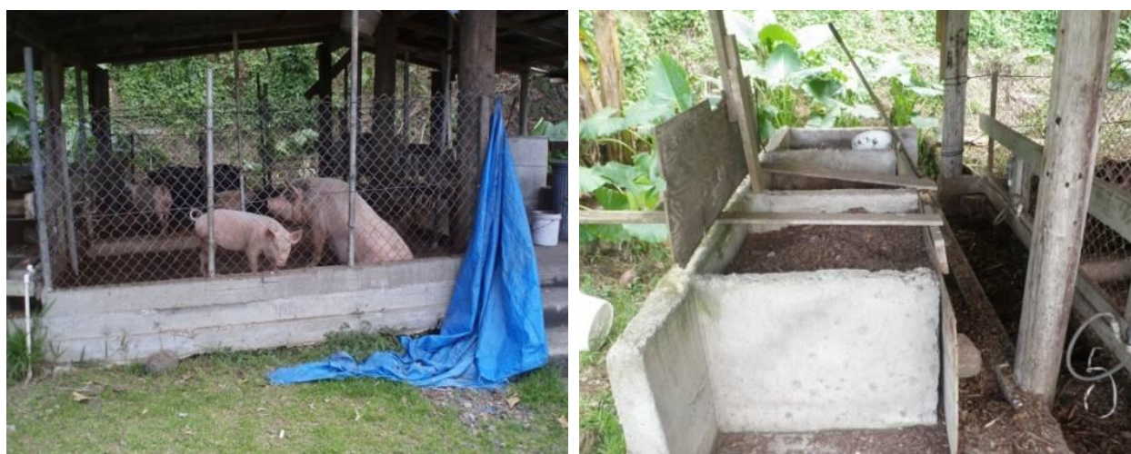
Figure 9. This dry litter piggery is a pen with a roof and sloped concrete floor. The waste is collected in a trench and then is composted with dry plant material such as wood chips or coconut husks.
