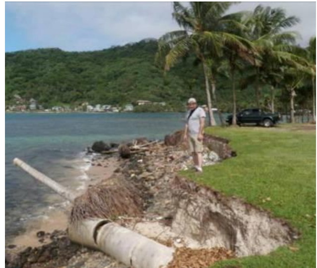
Figure 10B. Outfall of existing/historic storm drainage pipe
