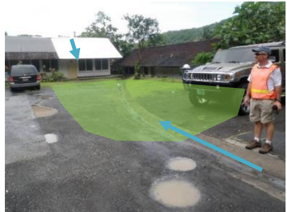
Figure 7A. Proposed location for small bioretention in upper parking lot. A portion of the parking lot is also proposed to be converted to permeable pavers.
