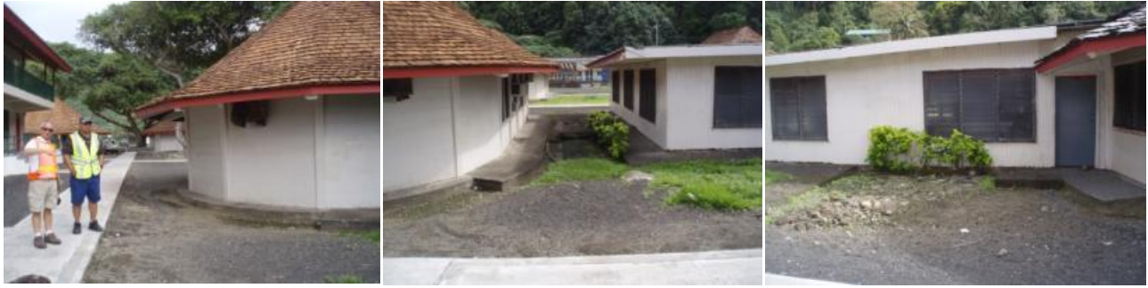
Figure 10C. Broken panorama of location of bioretention location 10B.
