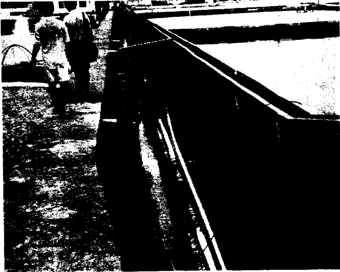
Figure B-3. Concrete-walled ponds at farm 1, away from the ocean. The central drainage canal separates the older ponds on the right from the newer ponds on the left. Seawater supply pipes are in the drain canal, and a water supply canal is on top of the older pond walls.
