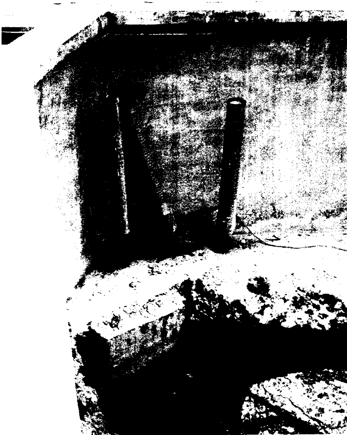
Figure B-19. Outlet pipes on a pond under construction near Tungkang.
