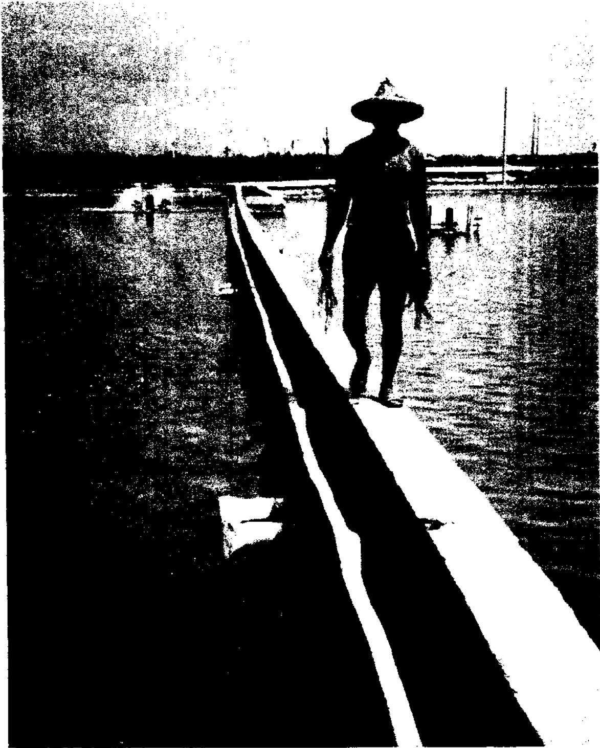
Figure B-10. Concrete wall at farm 9 with built-in water supply canal on top.
