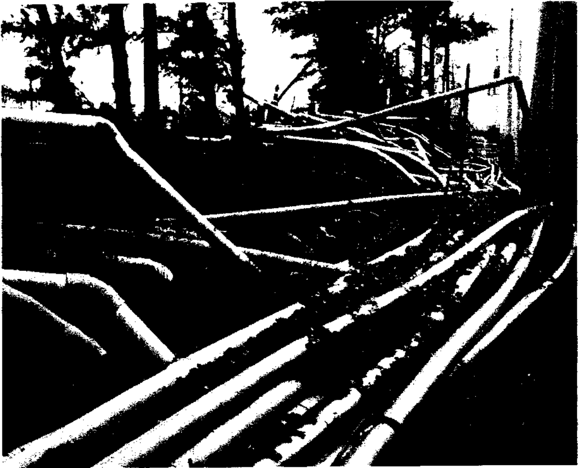
Figure 7. Seawater supply pipes leading from the wells near the ocean to many farms inland. Pipe diameters are typically 11 cm (4 to 5 inches).
