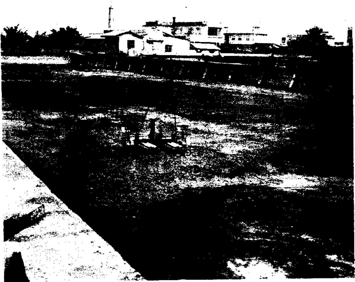
Figure B-5. Concrete-walled ponds at farm 2. Two 1 hp paddlewheel aerators are seen resting on the dried bottom.
