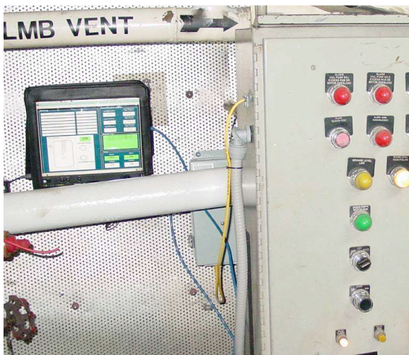
Figure 10: Real-time NILM monitoring CHT on the USCGC Escanaba .
