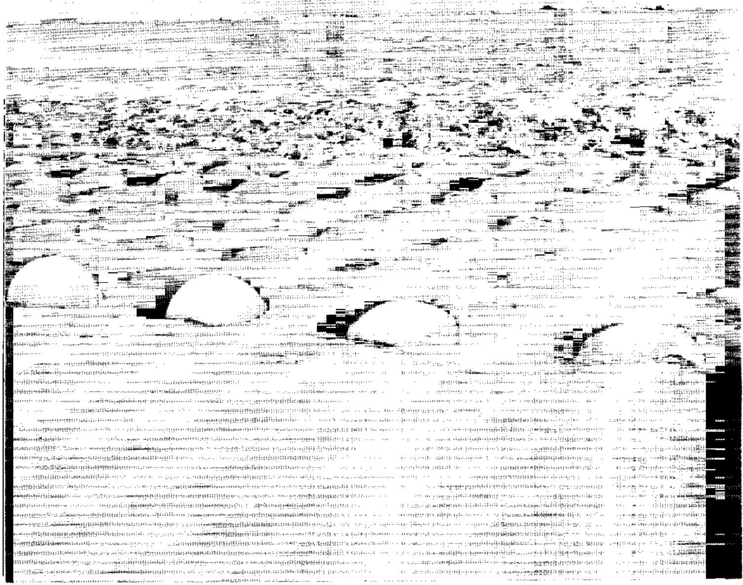
Boat wake attenuation through a section of a Tethered Float Breakwater, San Diego Bay.
