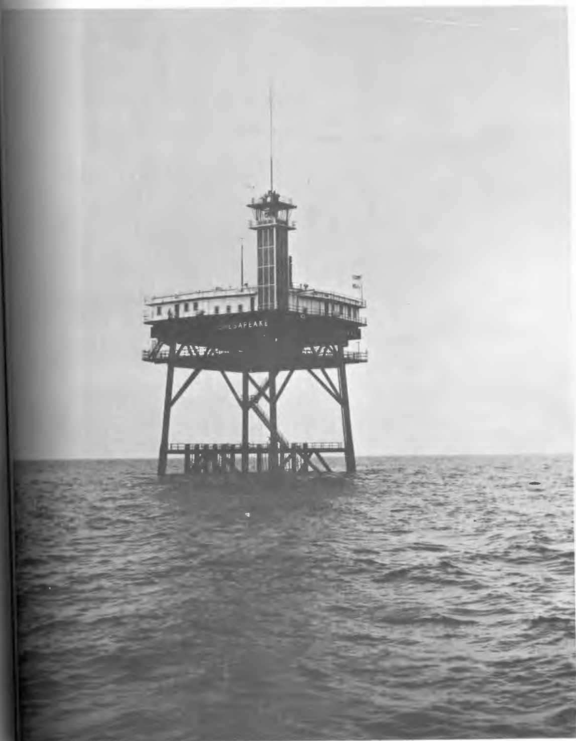
Figure 1. Chesapeake light tower.
