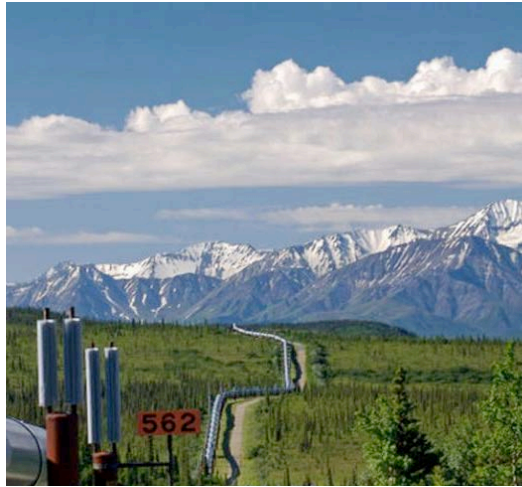
Fig. 3 Thermosiphons protect the trans-Alaska pipeline from permafrost damage. Source: http://www.eoearth.org/article/Permafrost
