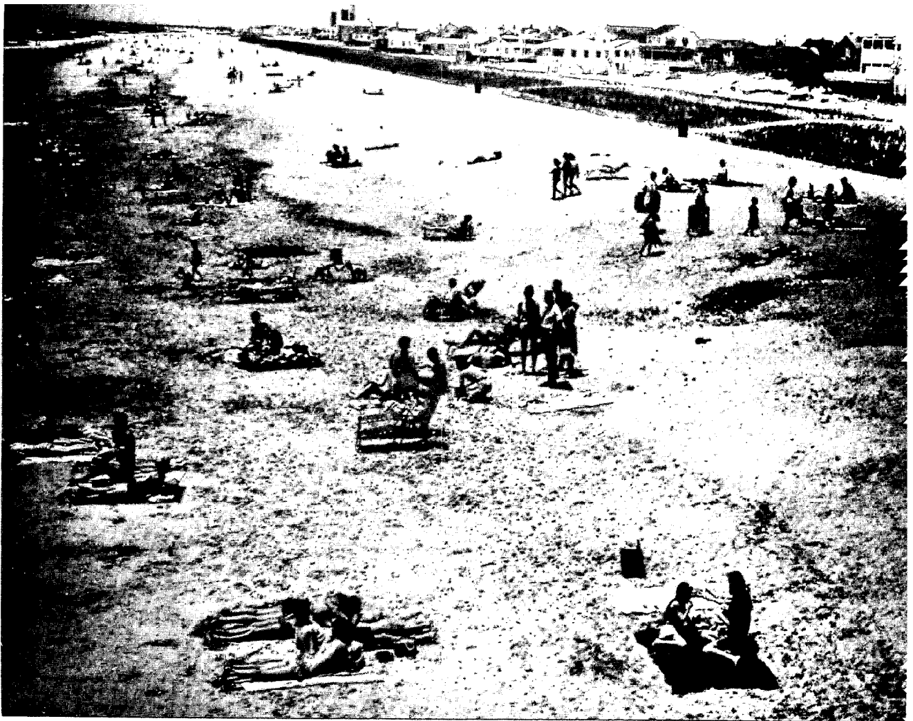
Figure 35. Wrightsville Beach, North Carolina, after completion of Beach Restoration and Hurricane Protection Project
