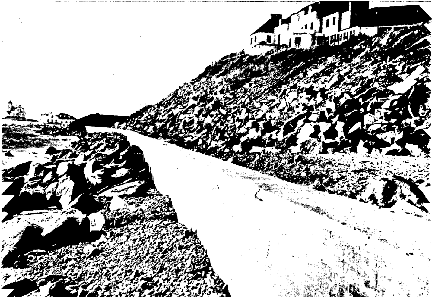
Figure 18. Vertical-face Concrete Seawall built 25 years ago at Watch Hill, Rhode Island. Seawall, combined with heavy rock riprap, protects the residence on hill at right. Photo from Portland Cement Association.
