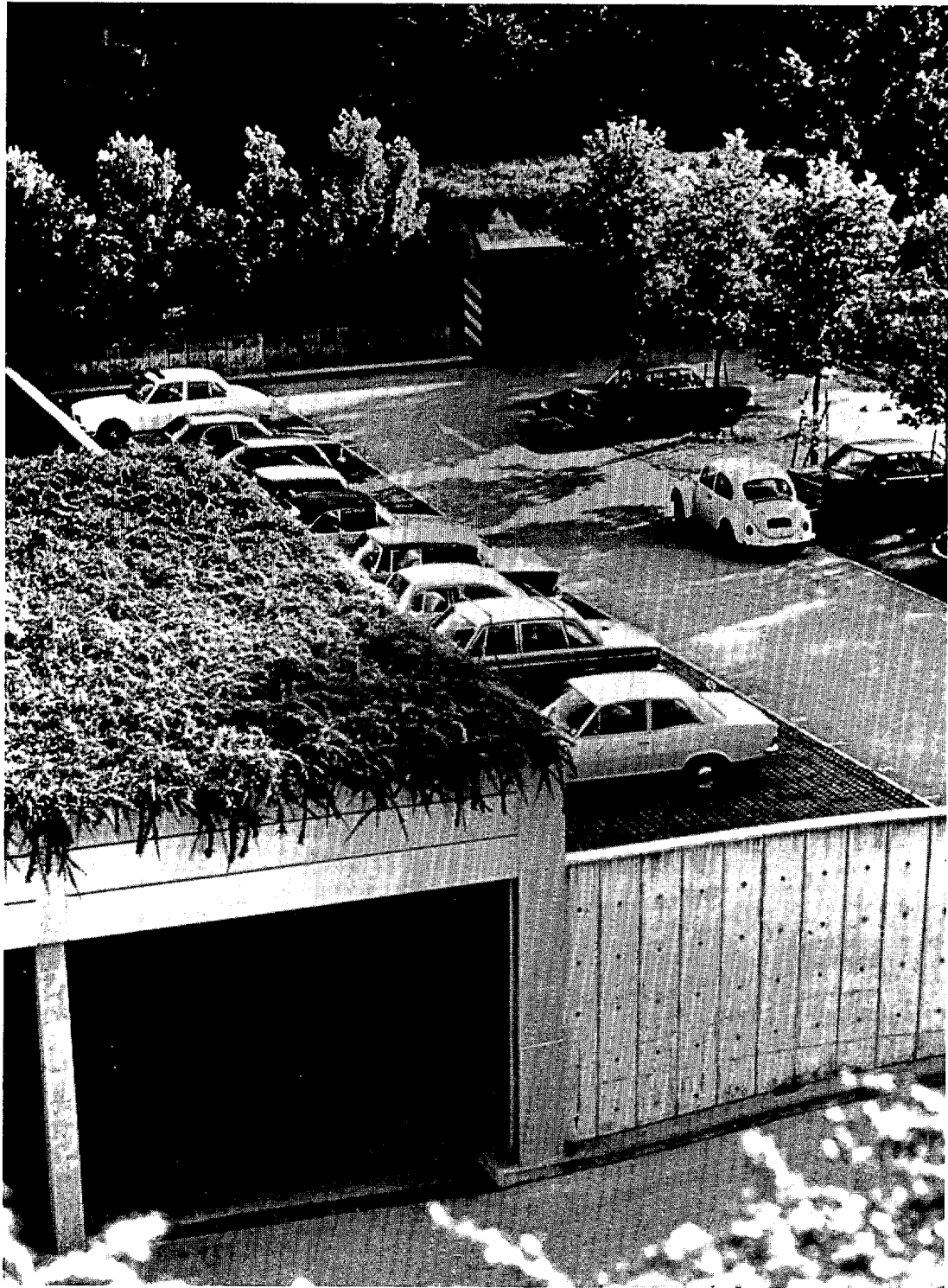
Porous grid pavers with grass cover and vegetated rooftop detention form a attractive and well-maintained design solution in Stuttgart, West Germany.
