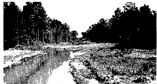
Typical surface flooding
