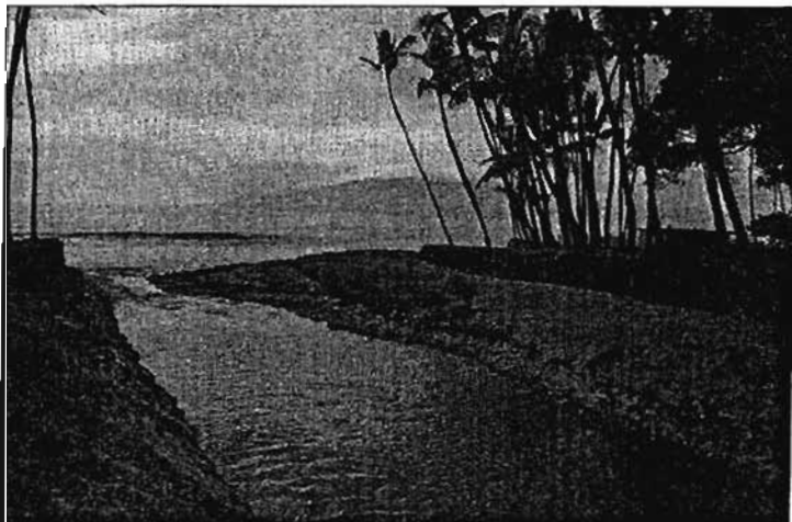
Figure 22. Formation of a sand bar or barrier at the stream outlet is one of the drawbacks with the design commonly used for stream channels. These channels work well to protect adjacent properties from flooding, but the standing water behind the sand bars often elicits complaints about noxious odors.
