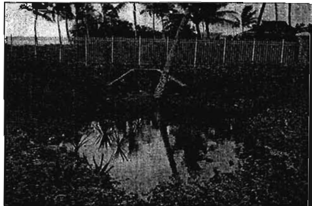
Figure 18. This attractively landscaped water holding pond was designed into a new development at Kai Ala Place. A series of landscaped depressions helps to retain flood waters and partially compensate for the fill and impervious surfaces that will increase runoff from the fully developed site.
