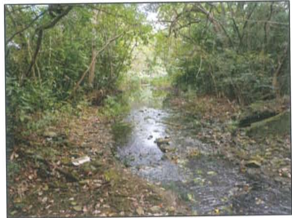
TR-35 culvert. USGS gauging station is upstream from here.
