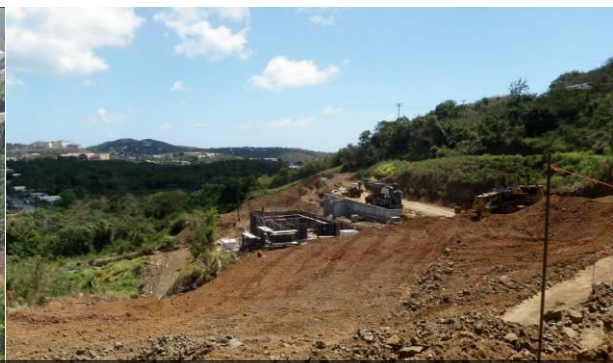
Grandview uses erosion control blankets and riprap to stabilize some slopes, but there remain acres of exposed soils and failing perimeter silt fencing that result in sedimentation downstream.
