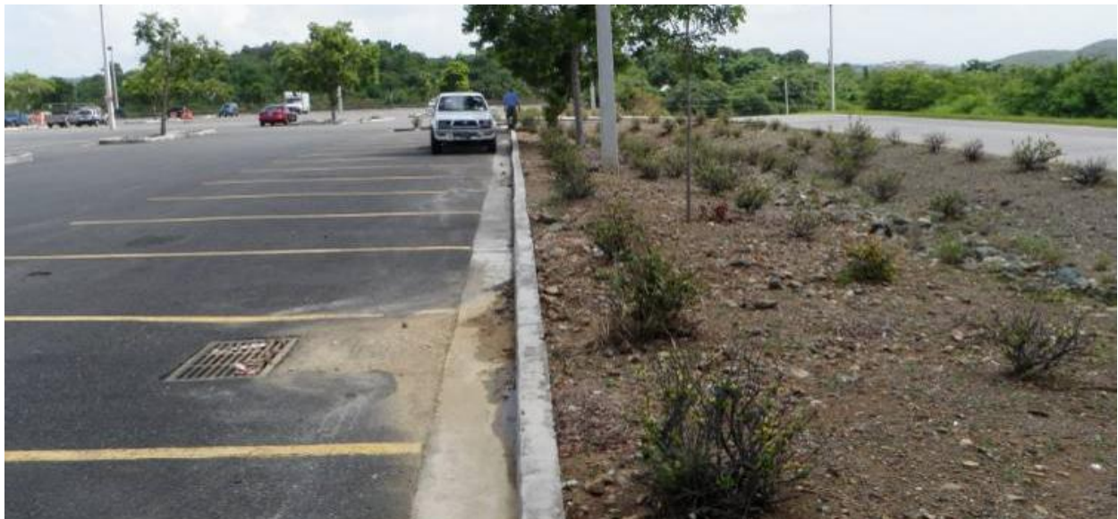
Retrofitting can help improve existing conditions. An easy fix at Home Depot is to block this inlet and allow parking lot runoff to flow into landscaping via curb cuts, allowing for plant uptake, infiltration, and filtering.
