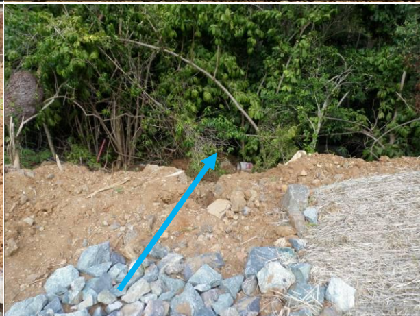
Outfalls discharge stormwater from Grandview roads and parking lots directly to the gut without any form of water quality treatment or flow detention.
