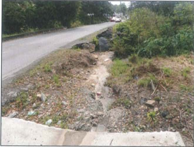
Concrete channel and scour downstream of culvert at TR-37.
