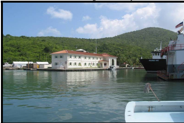
Coast Guard Building at Cruz Bay Harbor
