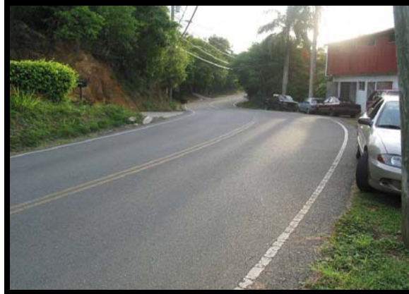
Narrow Highway 33 above Caret Bay
