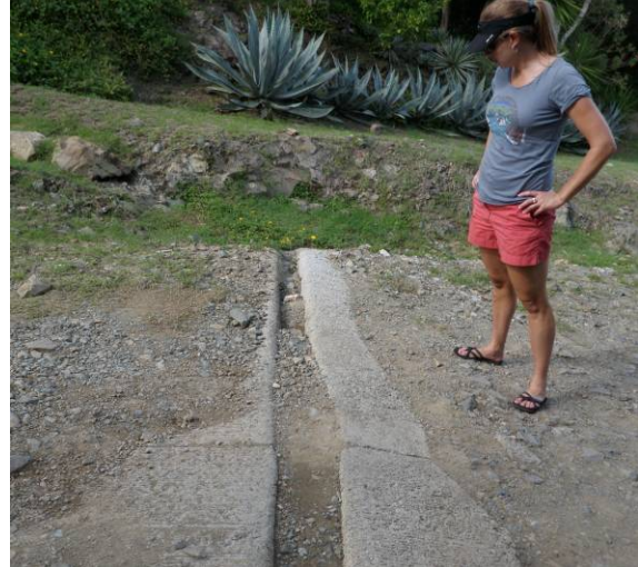
Figure 33. Open top-culverts have to be designed for maintenance access. The spacing should be wide enough to fit a narrow shovel. Top left and right photos here show clogged practices with reduced functionality. The grated cross-drain (bottom left) works on paved surfaces, and the grate can be lifted for easy cleaning. Be sure to provide outlet protection (bottom right) and remove deposited sediment on a regular basis.
