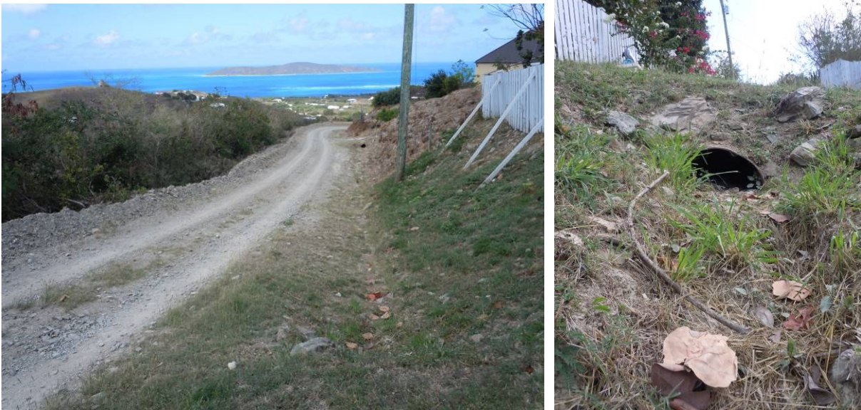
Figure 11. Coral Reef Trail in this area is very steep (left) with damaged/clogged driveway culverts (right).
