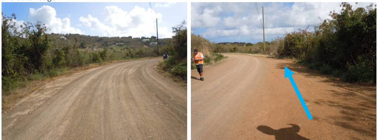
Figure 25. The entrance to Hibiscus Circle is wide and mostly flat, with some evidence of ponding along the outer edge.
