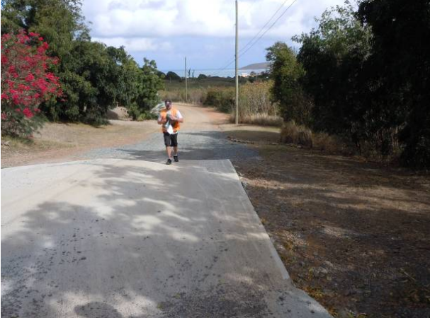
Figure 26. Some erosion is occurring at the edge of the paved intersection (left), and a manmade drainage path created to help runoff reach the eastern gut (right).
