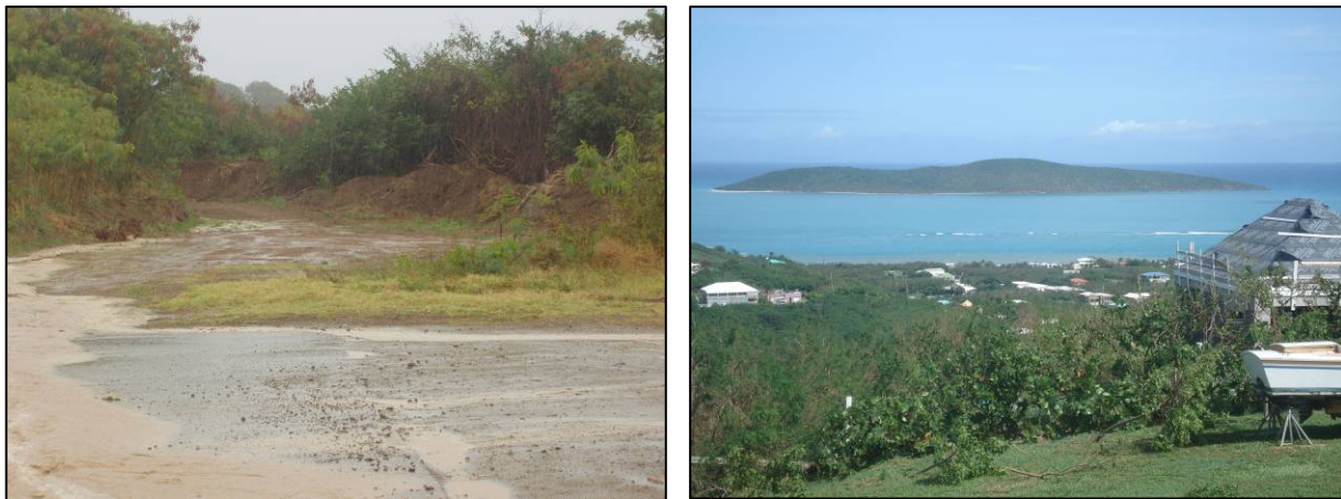
Figure 2. Sediment plume discharge into Solitude Bay, St. Croix, USVI (photo on right) from sources such as the Hope and Carton Hill road network (photo on left) after Hurricane Omar in 2008.
