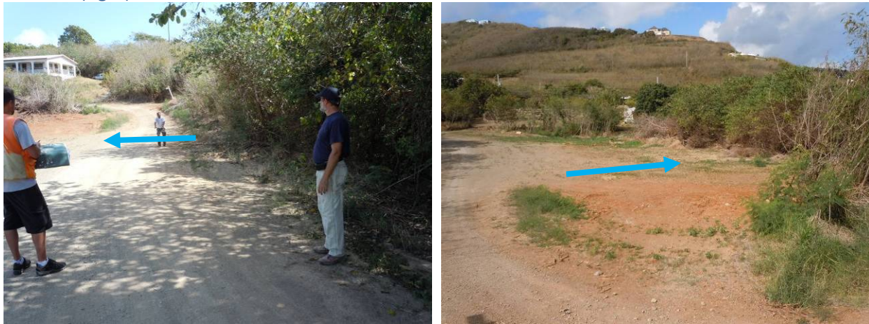
Figure 20. The gut flows over Yellow Cliff Trail at this location (left); the maintenance contractor has cleared the private lot in this area in an attempt to better accommodate gut flows to prevent flooding of the road (right). Flow arrows shown in blue.
