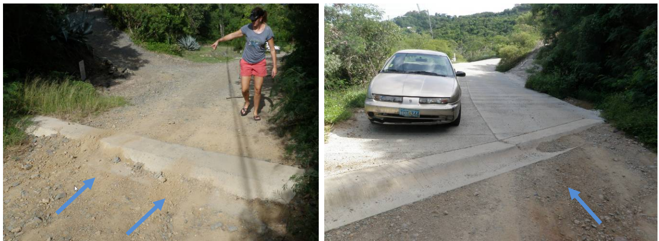
Figure 29. Proper angling and pitch of waterbar will help keep sediment from accumulating in swale
