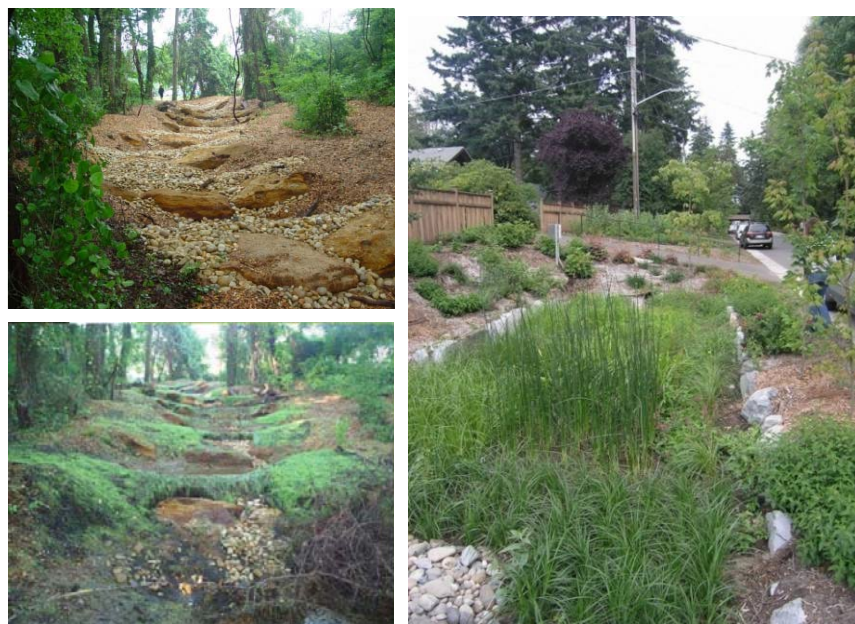
Figure 38. Photos showing stepped conveyance systems in channel from Anne Arundel County, MD (two photos on left), and a linear bioretention facility along a residential street in Seattle, WA (on right)
