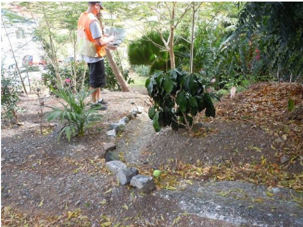
Figure 26. Some erosion is occurring at the edge of the paved intersection (left), and a manmade drainage path created to help runoff reach the eastern gut (right).
