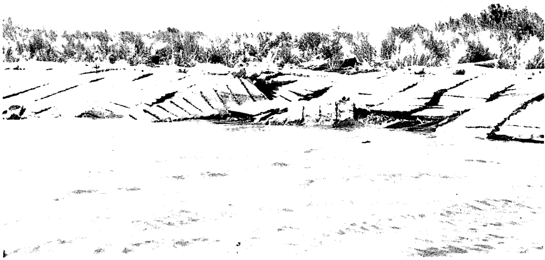
Figure 44. Photograph taken 27 March 1984 of failed test section 6, MRGO foreshore protection project.
