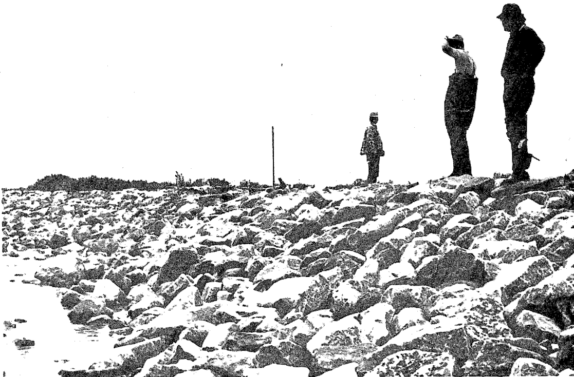
Figure 39. Photograph taken 27 March 1984 of test sections 1 and 2, MRGO foreshore protection project.
