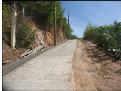
Photo 14: Marina Drive during paving.
