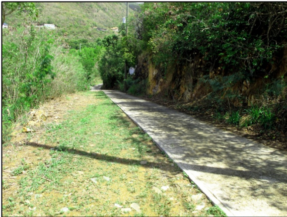
Photo 21: Completed Marina Drive paving.
