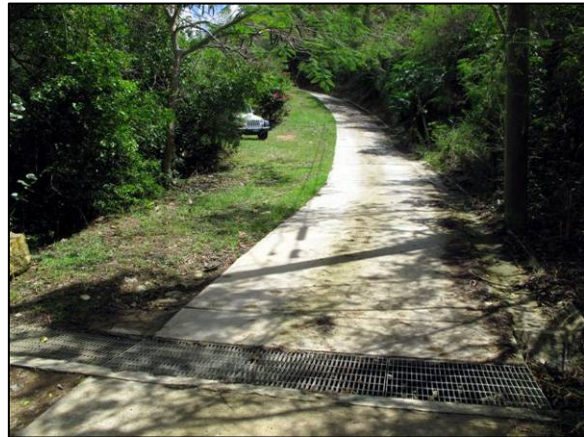
Photo 22: Completed Marina Drive paving and trench drain.
