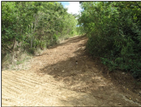
Photo 9: Z-Road during grading.
