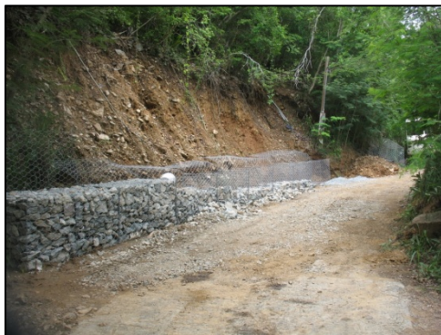
Photo 17: Cut-slope stabilization gabion basket installation.
