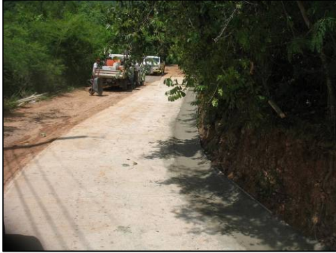
Photo 13: Marina Drive ditch paving.
