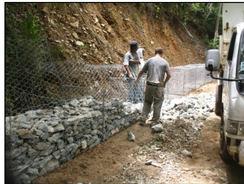
Photo 16: Cut-slope stabilization gabion basket stone installation.
