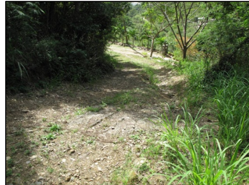
Photo 6: Z Road before construction.
