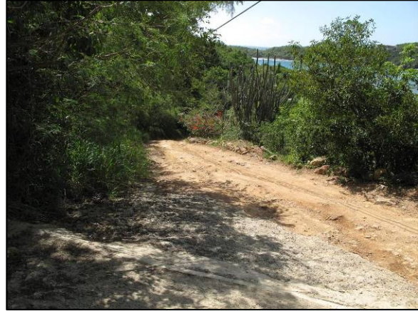
Photo 5: Unpaved road in Estate Fish Bay.
