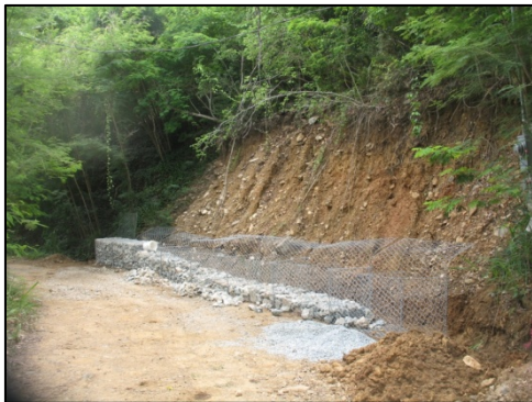
Photo 15: Cut-slope stabilization gabion basket installation.
