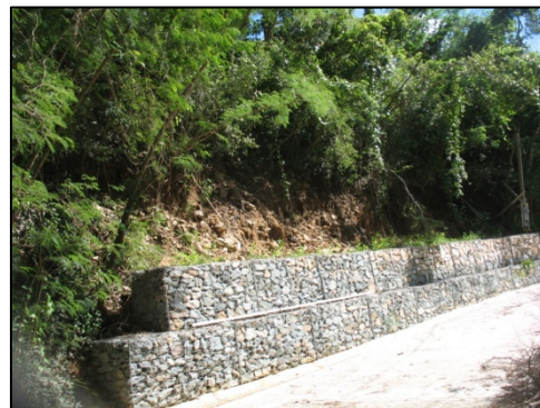
Photo 18: Completed cut-slope stabilization gabion basket installation.
