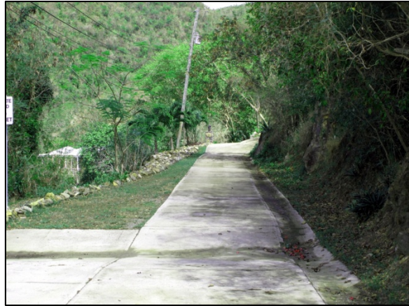
Photo 20: Completed Z-Road paving and concrete ditch and swale.
