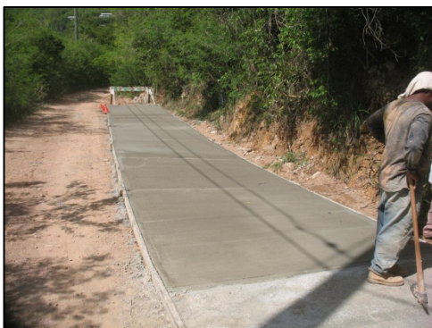
Photo 12: Marina Drive during paving.
