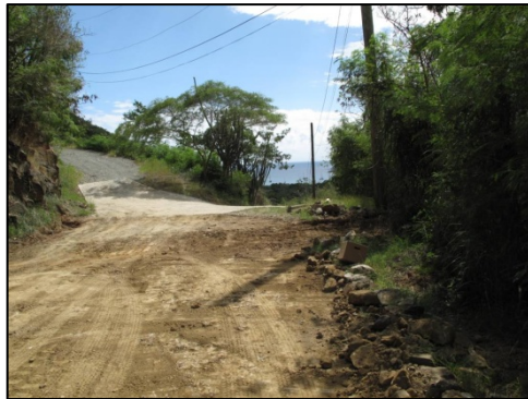
Photo 10: Z-Road during grading.
