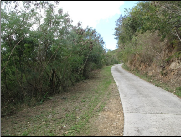
Photo 19: Completed Z-Road paving.
