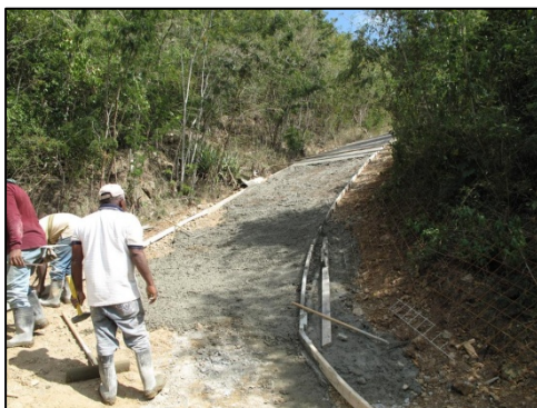
Photo 11: Z-Road during forming and paving.
