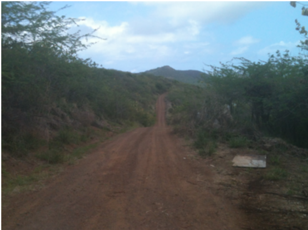
Figure 1. Illustrates one of the road areas for stabilization in Punta del Viento
