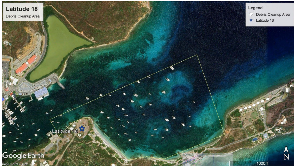
Figure 1. Debris Clean-up and Existing Structure Removal Area Shown outlined with a White Box (Image Provided by USACE).
