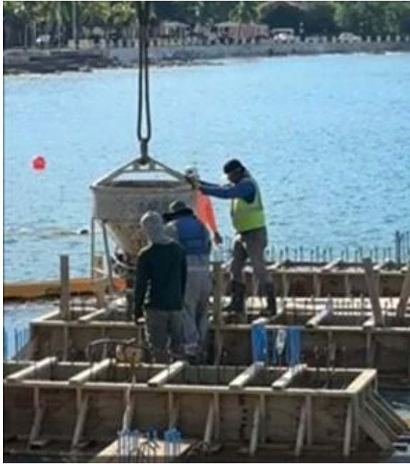
Figure 5. Example of pouring concrete with a specialized bucket.
