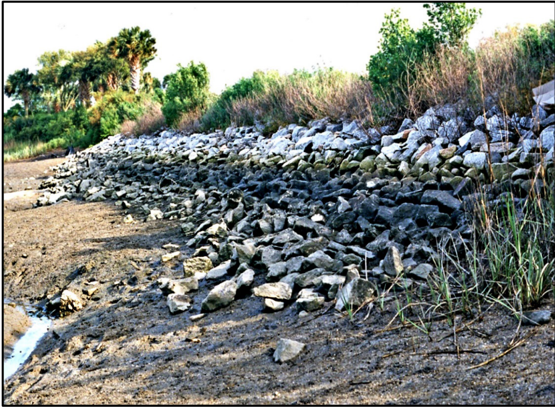
Figure 2.23: Sheltered Riprap with ESI rank of 8C.
