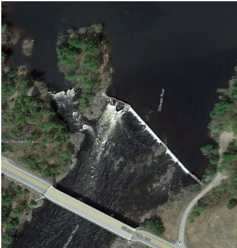
Figure 2. An overview of the Gilman Falls Dam, which is part of the Milford Hydroelectric Project. The dam is located on the Stillwater Branch.
