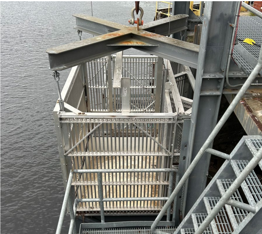
Figure 3. The new trap constructed in 2021 that can be placed at the exit of the Denil fishway.
