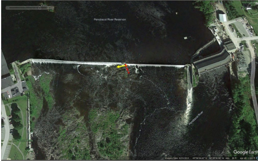
Figure 4. Schematic of proposed spill diversion wall (red dotted line – approximate location). Yellow arrow shows where, when the Obermeyer is lowered, some flow on the western side of the Obermeyer spills over the center ledges. Red line depicts approximate location of proposed flow diversion wall.
