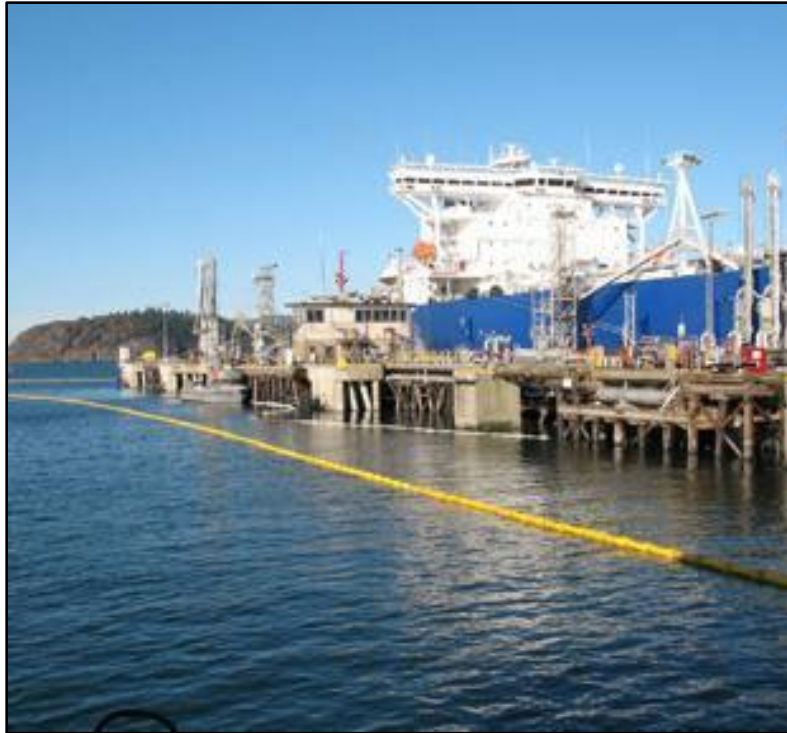
Figure 3.1-3. Booming: deployment of a floating barrier (seen in yellow) to contain marine spills and protect the environment
