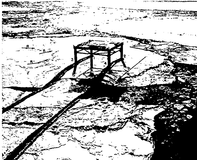
Test Platform at Middle Ground Shoal in Cook Inlet 1964-65 showing direction of ice movement A →, and rafted ice R → .
