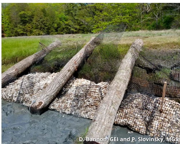
D. Bannon, GEI and P. Slovinsky, MGS Tensar GeoReef baskets tucked under installed logs and filled with shell. Excess crevices above the baskets were filled with coir bags and coir bags were installed along the remainder of the treatment. GeoReef basket lids were custom cut and twined closed with a UV-stabilized braid; coir bags were staked and twined using a double-cross pattern.
