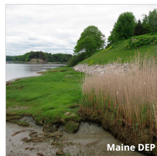
Maine DEP Project began in 2012 using a combination of hard and soft engineering: riprap at the toe of the slope and coir logs locked in place with helical anchors and secured with reinforced turf mats and native salt marsh vegetation. The existing vegetation was cut to ground. The slope was regraded, and geotextile material placed in combination with topsoil, erosion control mix, and native plantings. Biodegradable jute mat was used to prevent erosion while the vegetation established.
