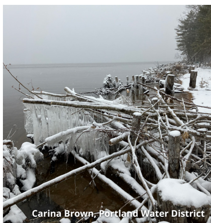
Carina Brown, Portland Water District Root wads, post-assisted wicker weaves, and brush aggradation bundle structures at Sebago Lake State Park addressing chronically eroding shoreline near the park's swimming beach area. Lake level is especially high from 2024 winter storms. These structures were designed to be out of harm's way from winter ice sheets.
