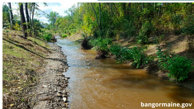
bangormaine.gov The City of Bangor Capehart Brook Restoration is being completed in accordance with the watershed-based plan for Arctic Brook. Beginning 2021, Phase III included this in-stream habitat improvement designed to increase in-stream velocities, improve habitat with the addition of coarse substrate and tree root wads, and restore flood plains.
