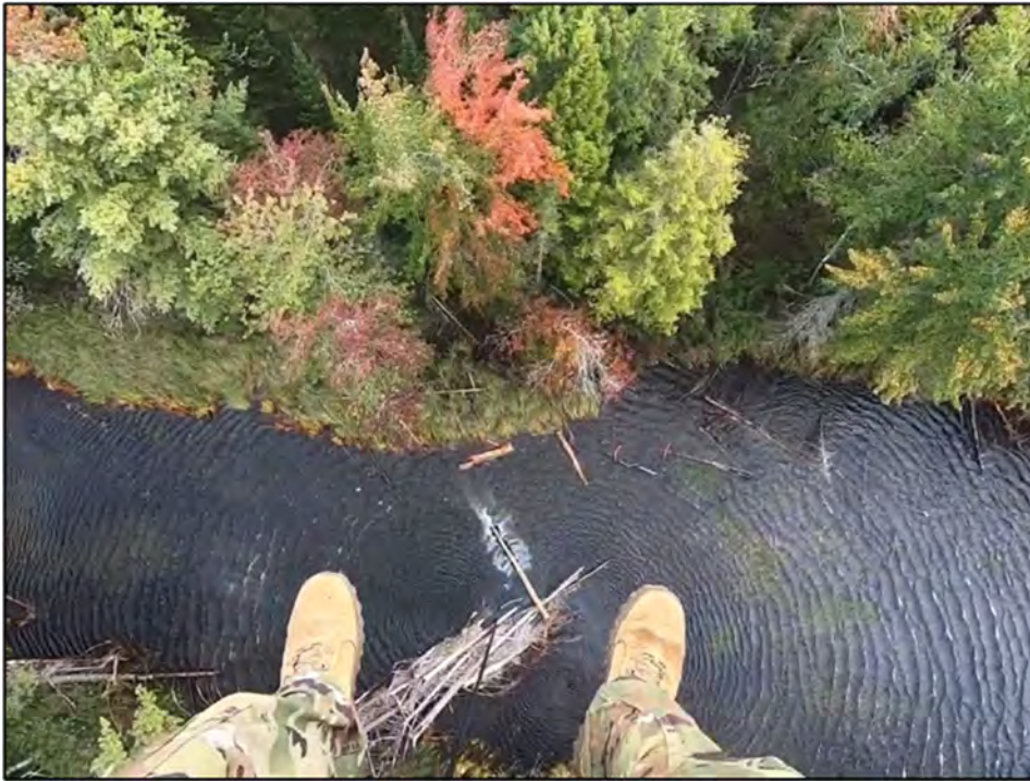
Figure 3.3.4. Releasing a load of large wood at the drop site as seen from the UH-60 helicopter crew chief's perspective, Narraguagus River, 2024. Photo credit: SFC Joseph Leclair.
