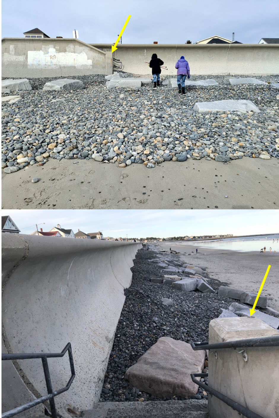
Figure 2-6: Example of a location where the seawall is too high to place a station marker (the seawall shown above is at North Beach, NH). In this case, a staircase at the base of the wall provides a good alternative to place a marker (see yellow arrow in bottom figure, which is pointing to a black mark on the corner of the concrete staircase). As seen in the lower figure, there is also enough space behind the edge of the wall to create a line-of-sight with the horizon for the first measurement.
