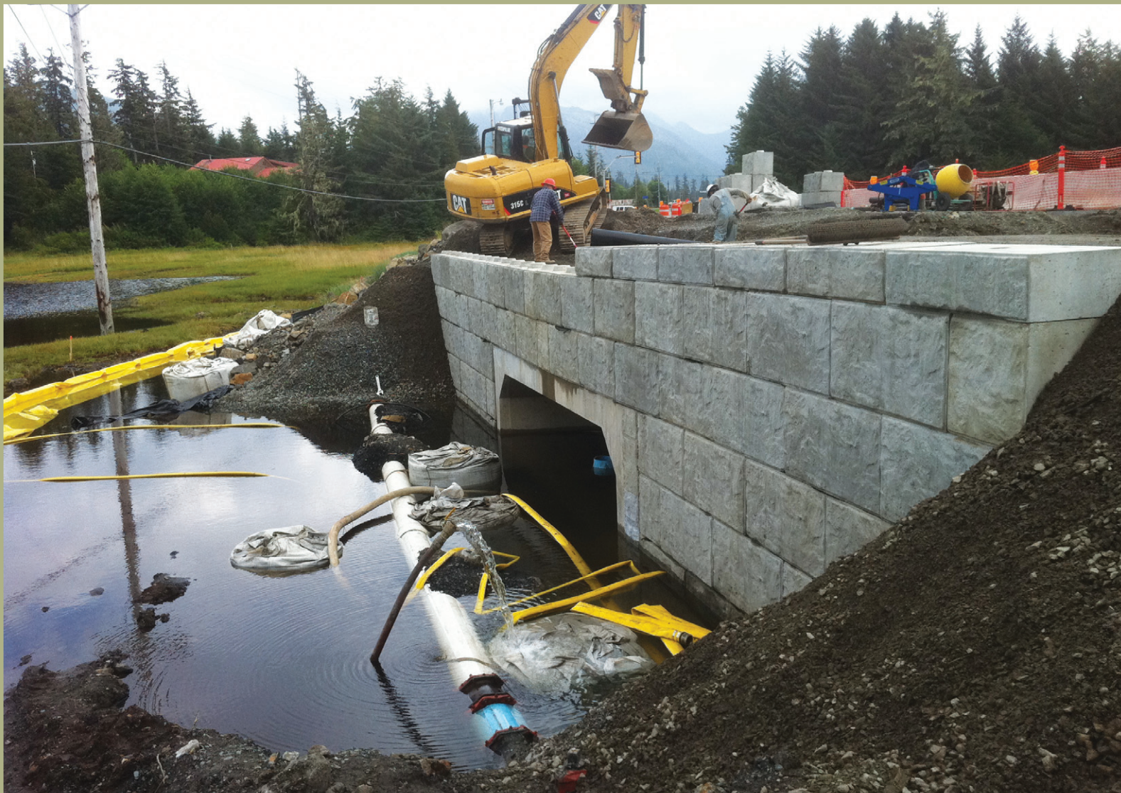
Construction of a larger culvert at the Klawock Highway. © Rob Bosworth, TNC
