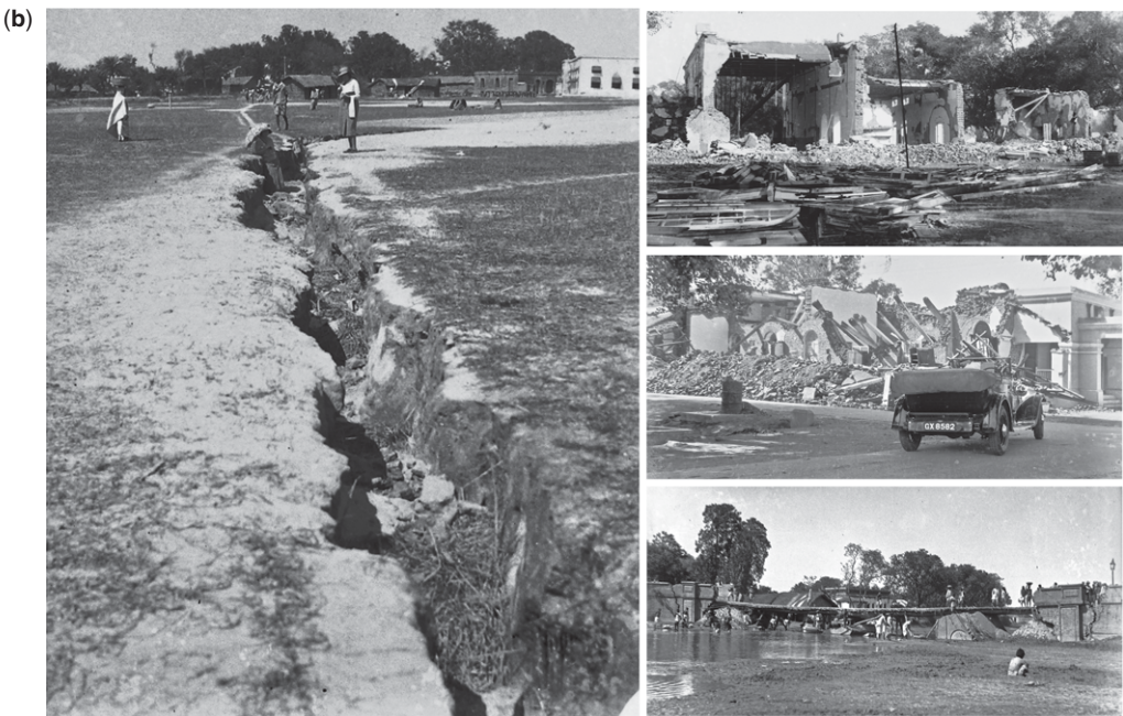
Fig. 20. Continued. (b) Scenes from the ‘slump belt’ of the Bihar province of India after the 1934 Bihar/Nepal earthquake. Sitamarhi (left at 26.58° N, 85.48° E), was long considered close to the epicentre of the 1934 earthquake. A typical fissure was 80 m long, 2.5 m wide and filled with sand to within 1 m of the top (Dunn et al. 1939, p. 149, and p. 210). Extensive lateral spreading and sand venting occurred during liquefaction of sediments in the Ganges Plain south of the rupture.
