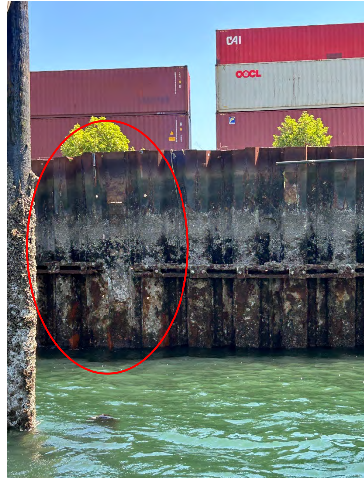
Port of Seattle's North Terminal 30, vertical sheet pile bulkhead located in deeper water. Note bulging, outward failure of bulkhead (red oval). No structural maintenance in more than 80 years.
