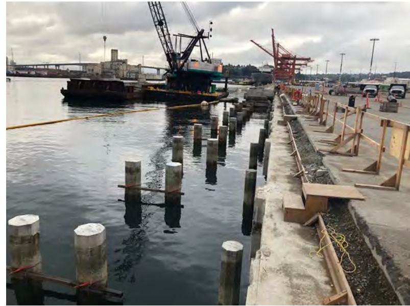
Port of Seattle's Terminal 5 during construction in 2019, illustrating octagonal concrete structural piling before pile cap and stringer installation.
