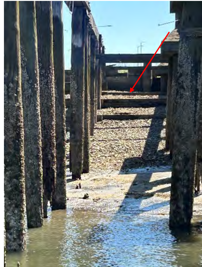
Port of Seattle's South Terminal 25, top-of-bank bulkhead (red arrow), with stepped series of toewall bulkheads. No maintenance in past 90 years.
