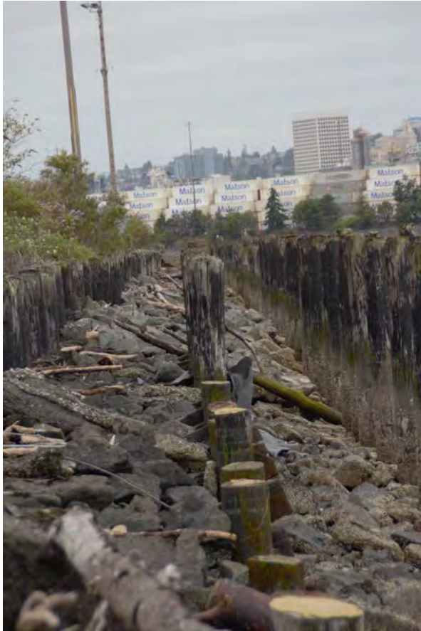
Port of Tacoma's North Intermodal Yard, step bulkhead with conventional armor and rubble-strewn slope. Aerial images indicate it was constructed between 1950 and 1973. Some of the creosote piling have been cut, but there has been no other measurable maintenance for at least 50 years.
