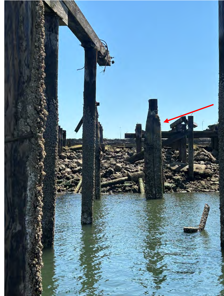
Port of Seattle's Southwest Terminal 25, illustrating common pile repair (red arrow). Pile was wrapped and pumped with grout. In this instance, the repair is approximately 45 to 50 years old. Meanwhile, portions of the surrounding 80-year-old timber pier have failed/collapsed.
