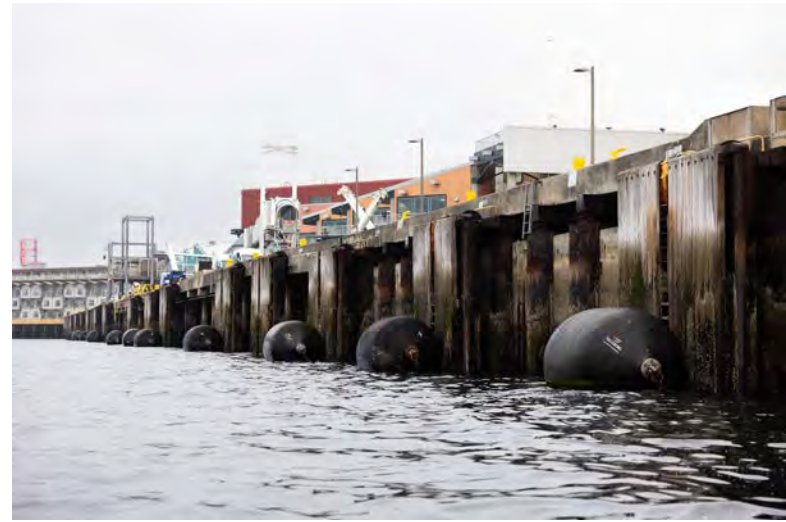
Port of Seattle's Pier 66 cruise terminal, with steel piling and timber- and rubber-bladder fender system. Steel piling was installed 2000 with no meaningful maintenance since installation.
