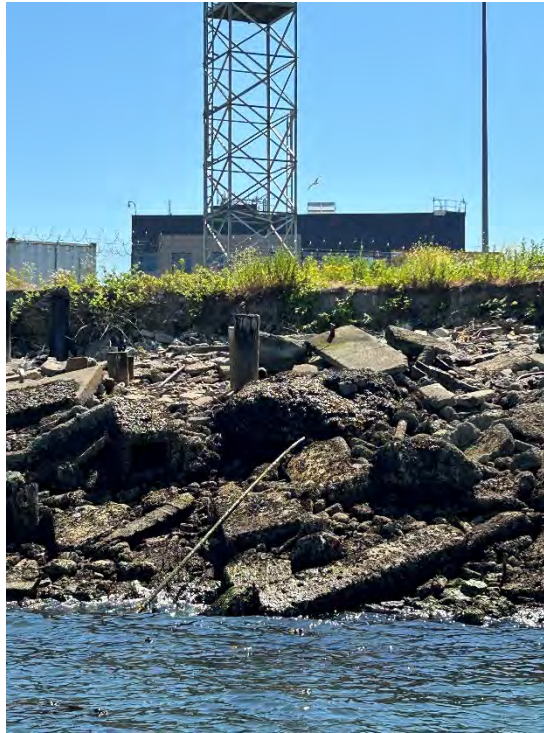
Duwamish Waterway shorelines with no measurable maintenance in the last 85 years.
