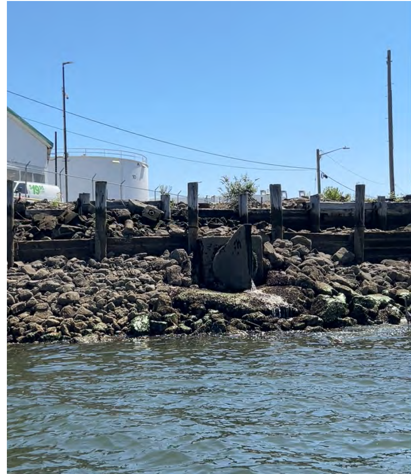
West Waterway, Harbor Island outfall, illustrating a double rank, creosote bulkhead and rock armor protection. Outfall structure has not been improved in past 90 years, except for the installation of "duck-bill" tide-gate, to replace a failed hinged, flap-gate.
