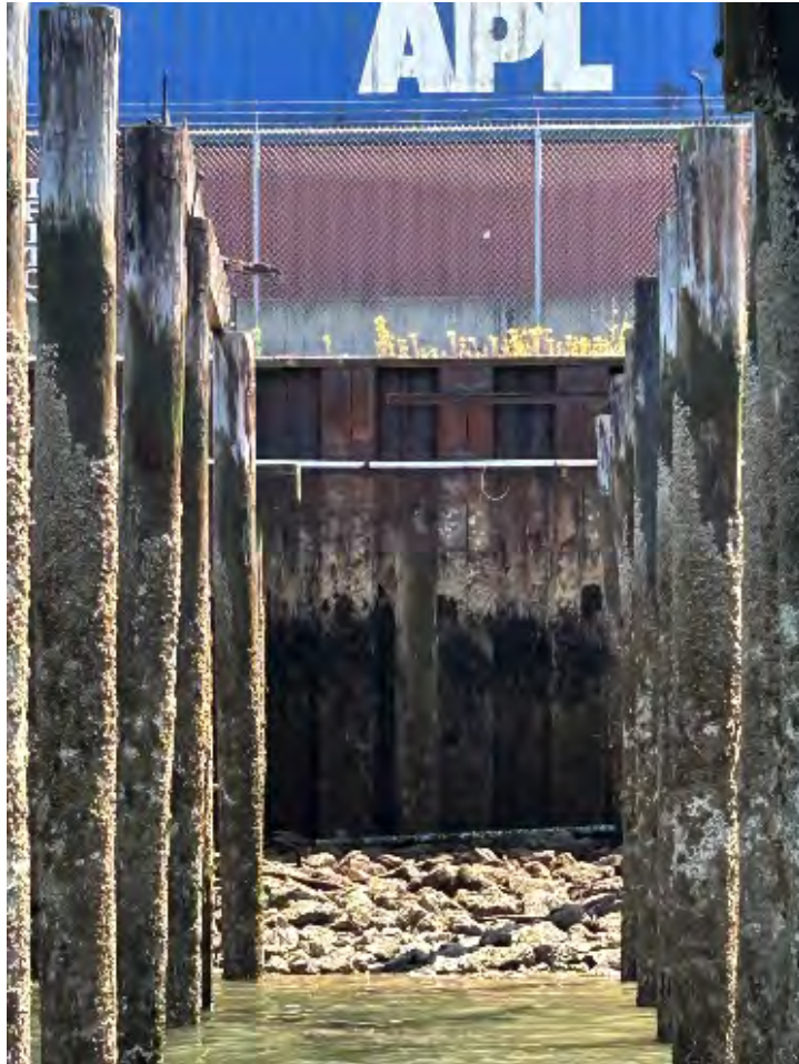
Port of Seattle's North Terminal 30, toewall is at the base of vertical sheet pile bulkhead and riprap is downslope of toewall. No measurable maintenance in past 80 years.
