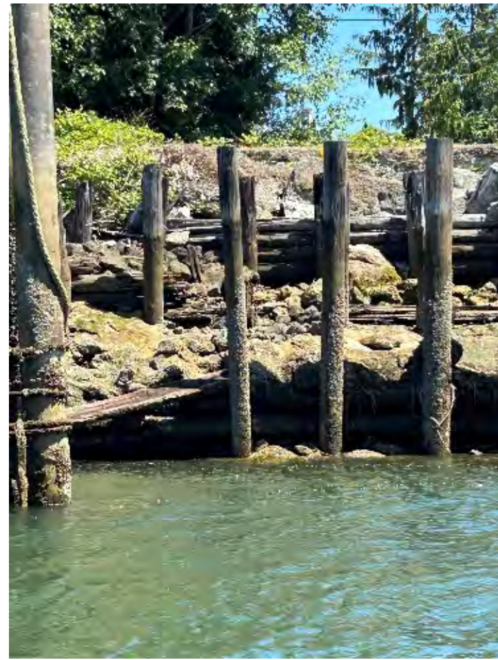
Upper and lower bulkhead, with latter functioning as a toewall. Note rock armor between bulkhead and toewall. No measurable maintenance in past 85 years.
