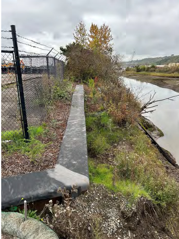
Port of Tacoma's Parcel 86 vertical bulkhead, installed 2020. This bulkhead protects an environmental cap from slope erosion. Future maintenance of this bulkhead will ensure the environmental cap is stable; thus, its maintenance is protective of the environment.
