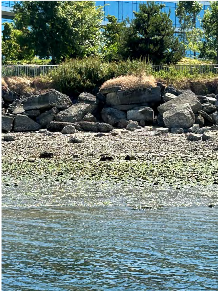
Northeast Elliott Bay, featuring heavy granite armor unimproved for more than 100 years. Armor is slumped with smaller material/sediments mobilized from subgrade behind the armored slope, littering intertidal area in the foreground.
