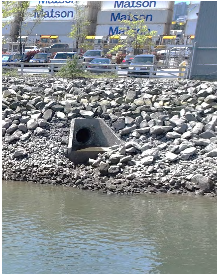
Sitcum Waterway 36-inch outfall and spillway installed 46 years ago. Maintenance consists solely of marine debris removal. No improvements to the concrete spillway since installation. Surrounding slope was re-stabilized in 2014.
