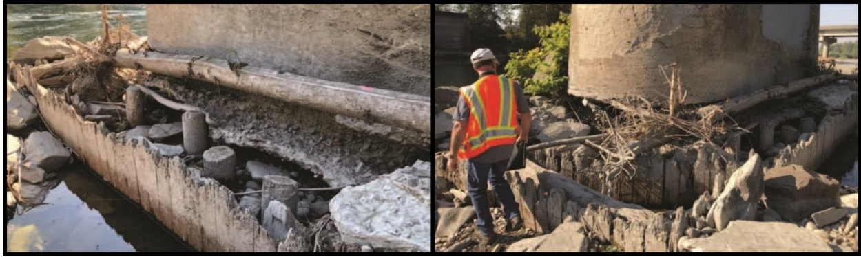
Figure 2. Photographs of Haller Bridge Pier 4 damage. The left image shows the north side of the pier, looking southeast (upstream). The right image shows the upstream end and north side of the pier, looking west (downstream) (Adapted from Figure 3 in Jacobs 2021a).
