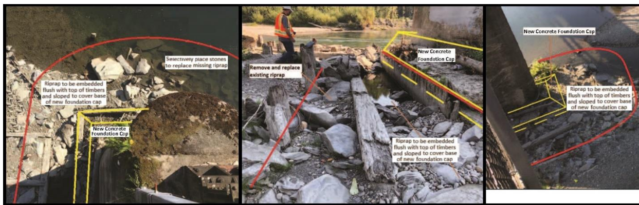
Figure 5. Photographs of Pier 4 showing the proposed concrete foundation cap in yellow and the riprap areas outlined in red (Adapted from Figures 5 in Jacobs 2021a).
