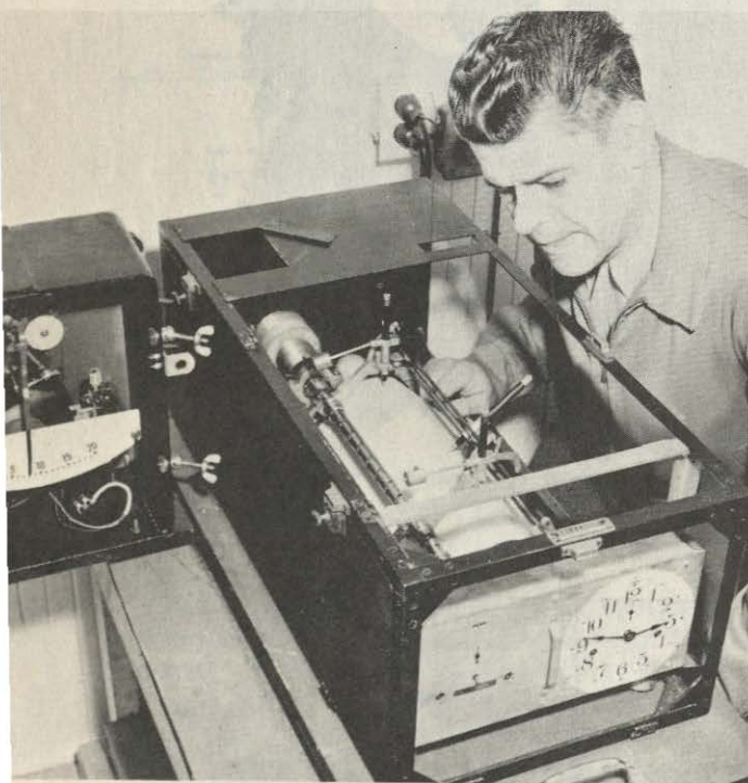
Recording mechanism of standard tide gage. (National Ocean Survey)
