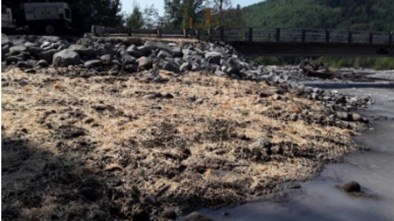
Figure 3. Photo upstream of emergency repairs after seeding and mulch was applied (Forest Road 7810 MP 0.1 Repairs Project BA).
