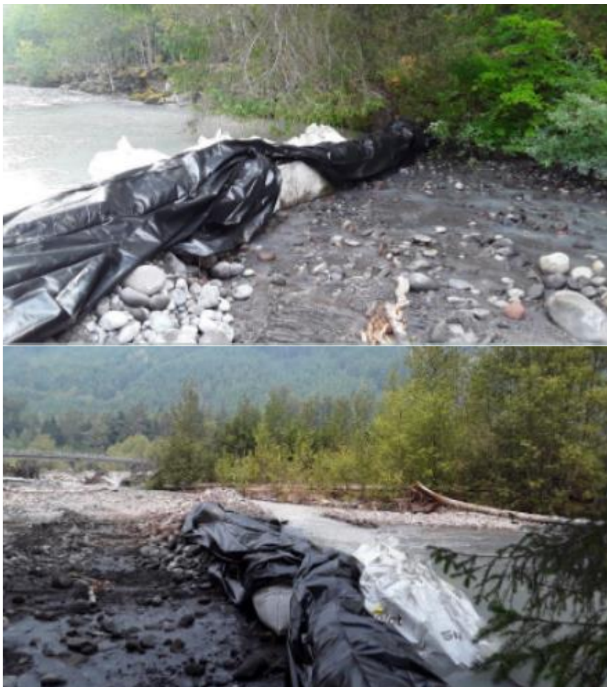
Figure 1. Photos of stream diversion for the emergency bridge repair (Forest Road 7810 MP 0.1 Repairs Project BA).
