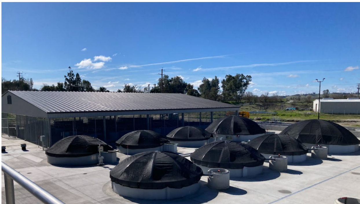
Figure 5. The new Salmon Conservation and Research Facility (SCARF) near Friant Dam. Shown in the picture are circular tanks (20 and 30 feet in diameter) that will house: adult broodstock raised and used for spawning (tanks within covered structure in background of photo), and juvenile salmon produced for release into the SJRRP Area (net-covered tanks in forefront of the picture). Photo Credit: NOAA Fisheries.
