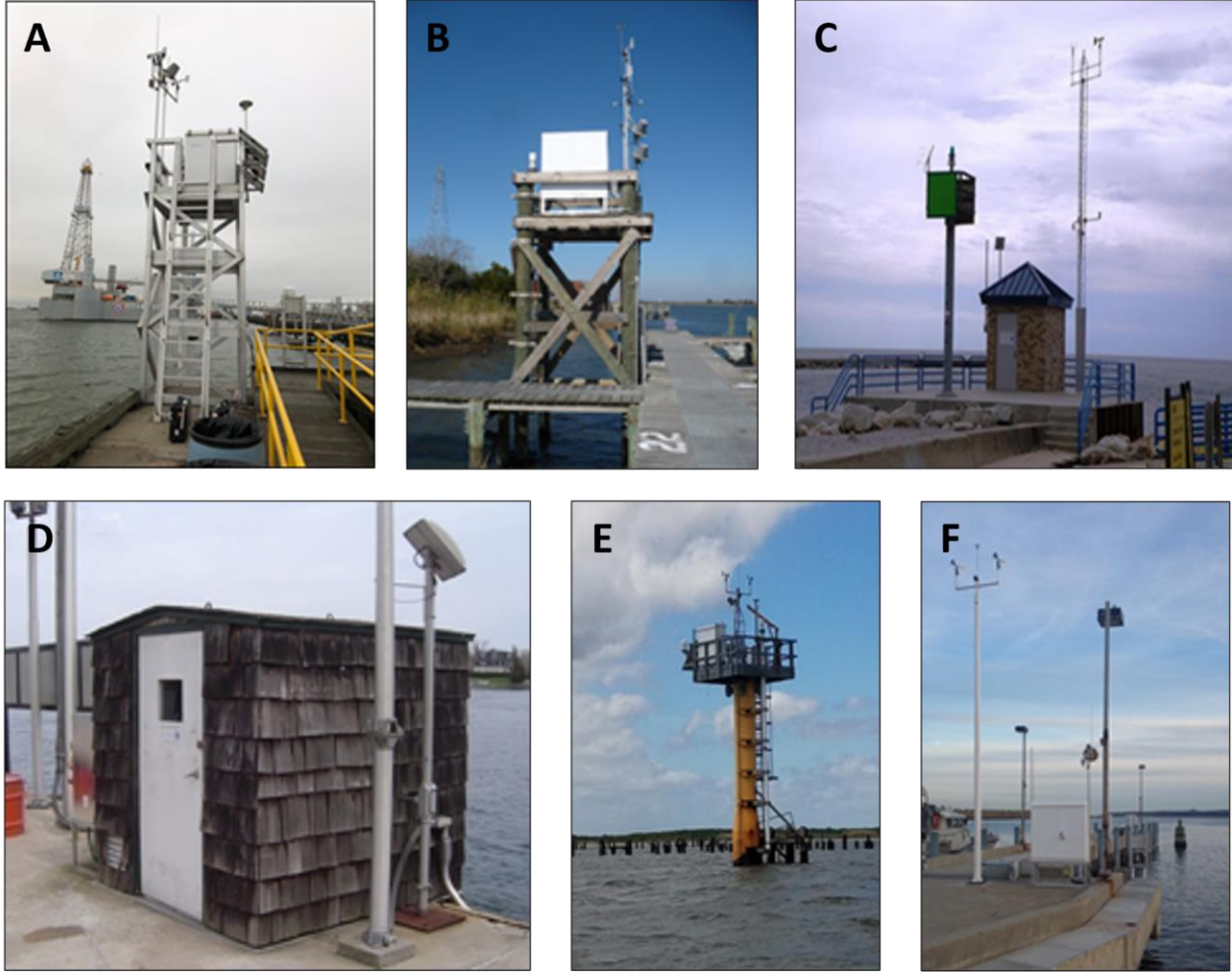
Figure 5. Examples of National Water Level Observation Network (NWLON) stations at Galveston Pier 21, TX (A); Apalachicola, FL (B); Great Lakes station with a stilling well at Holland, MI (C); Great Lakes station at Alexandria Bay, NY (D); Single Pile Instrumentation Platform (SPIP) station at Shell Beach, LA (E); and the station at Sandy Hook, NJ (F).
