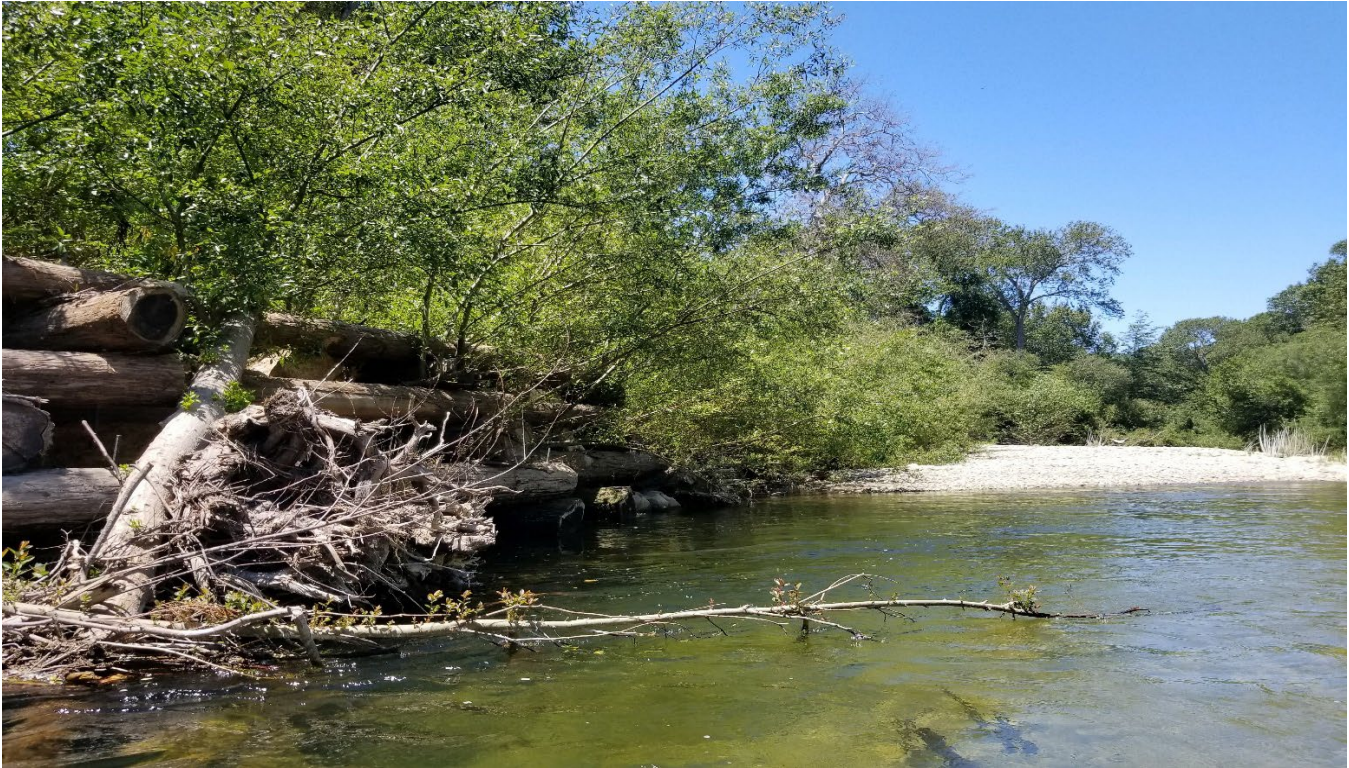
Figure 7. Rancho San Carlos bank stabilization/fisheries enhancement project after 5 years. Source: MPWMD 2023
