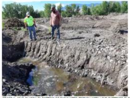
STAGE 1: MUD SLURRY IN BOTTOM OF EXCAVATED TRENCH WITH LIVE CUTTINGS PLACED WITH BOTTOM END EXTENDING BELOW GROUNDWATER.
