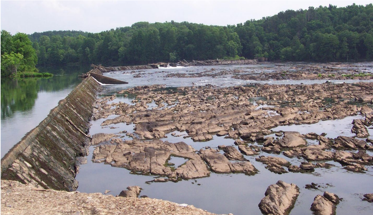
Figure 11. Shoal Habitat Below ADD During Low Flow Conditions (Photo Credit: E. Bettross, GADNR)
