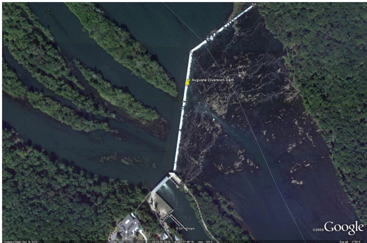
Figure 5. Augusta Diversion Dam. (© 2018 Google)
