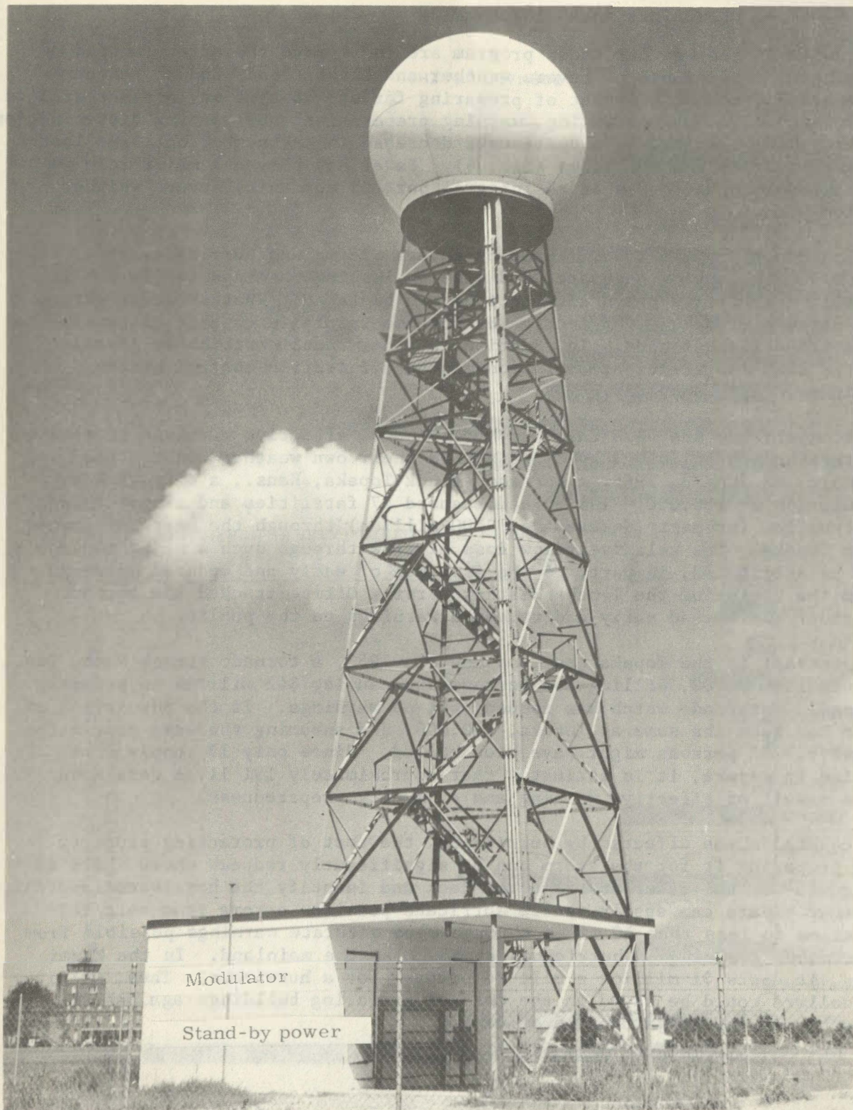
Figure 3.--WSR-57 installation at Charleston, S.C., showing tower, radome and building housing modulator, and auxiliary power.
