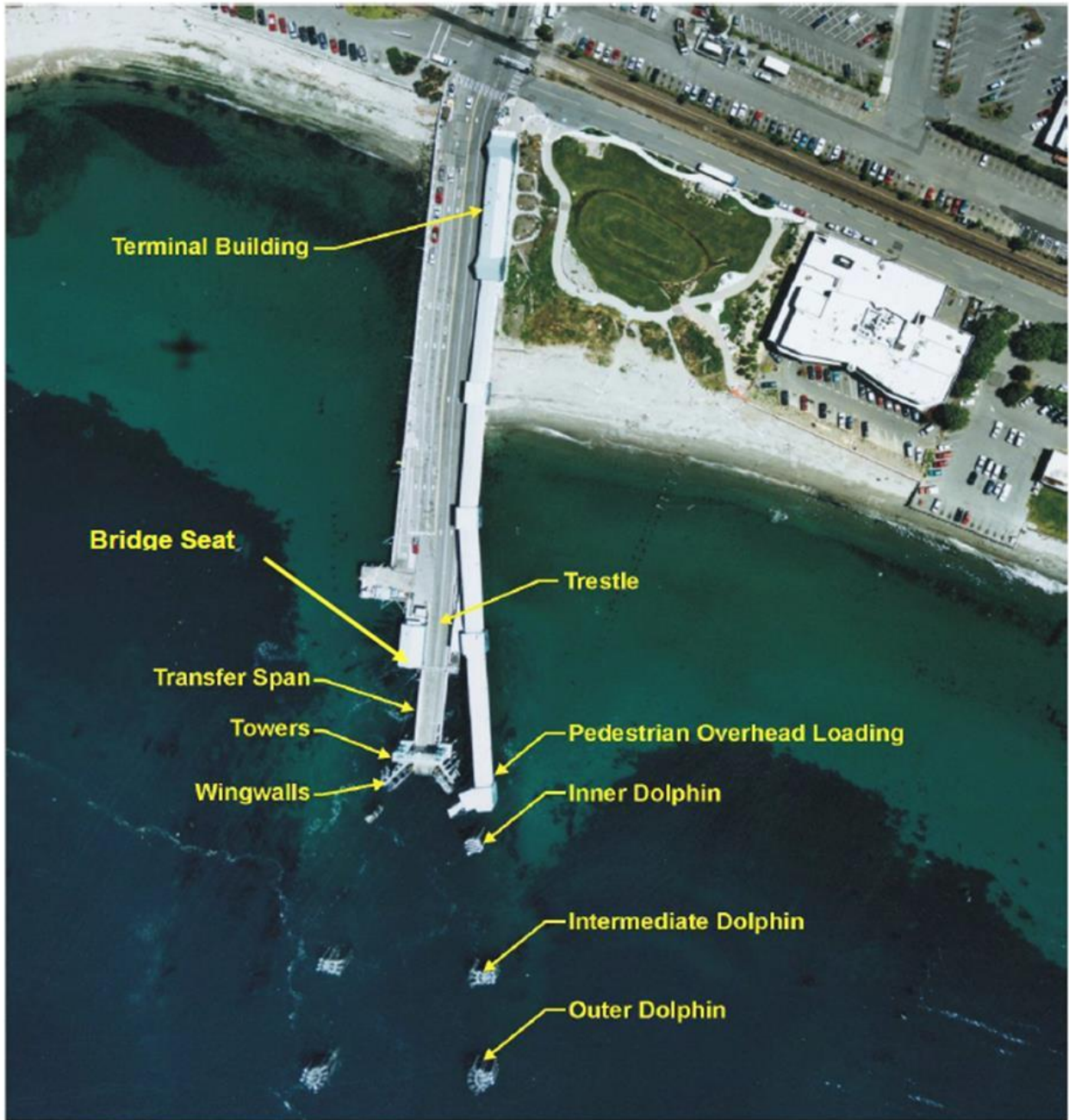
Figure 2. Structures commonly found at a ferry terminal
