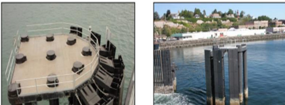
Figure 5. Typical fixed dolphins. Photos from WSF Terminal Design Manual, M3082.5, April 2016
