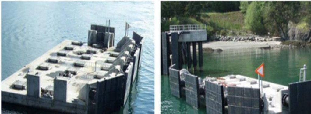
Figure 3. Typical floating dolphin. Photos from WSF Terminal Design Manual, M3082.5, April 2016.
