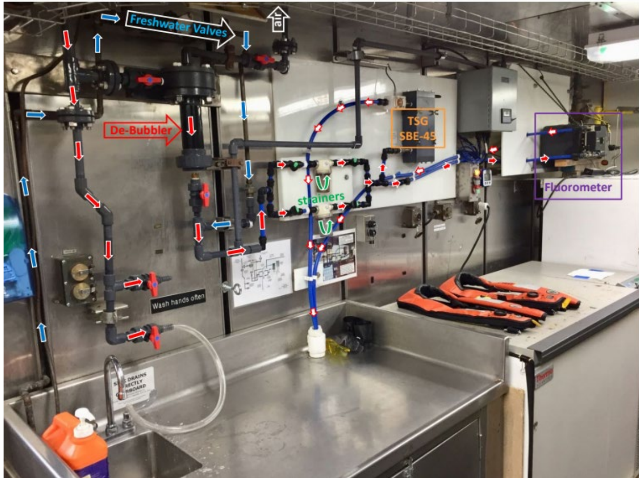
Figure 4. Flow diagram of Scientific Seawater System components in the wet lab, including the TSG. Photo: CST Wilkins.
