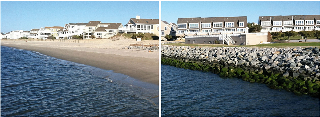
Fig. 2. Typical structural characteristics of the beach (left) and riprap (right) shorelines sampled
