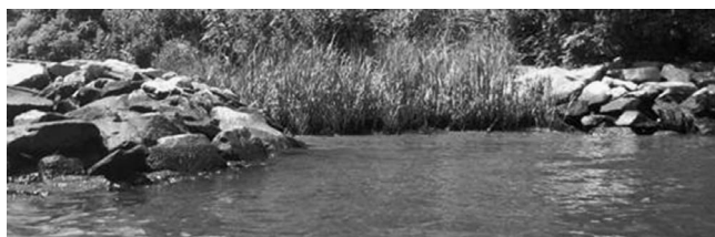
Figure 5. Marsh sills function as low profile stone breakwaters that are used to protect the created or enhanced fringe marshes from wave energy. Some designs have openings or gaps in the sill to allow for the exchange of tidal flow and to provide marsh access for marine animals. Marsh sills are typically constructed at MLW and then backfilled to create a suitable grade for marsh vegetation. The top of the sill is usually near MHW to provide the maximum protection while still enabling exchange of tidal water (Duhring, 2008b).
