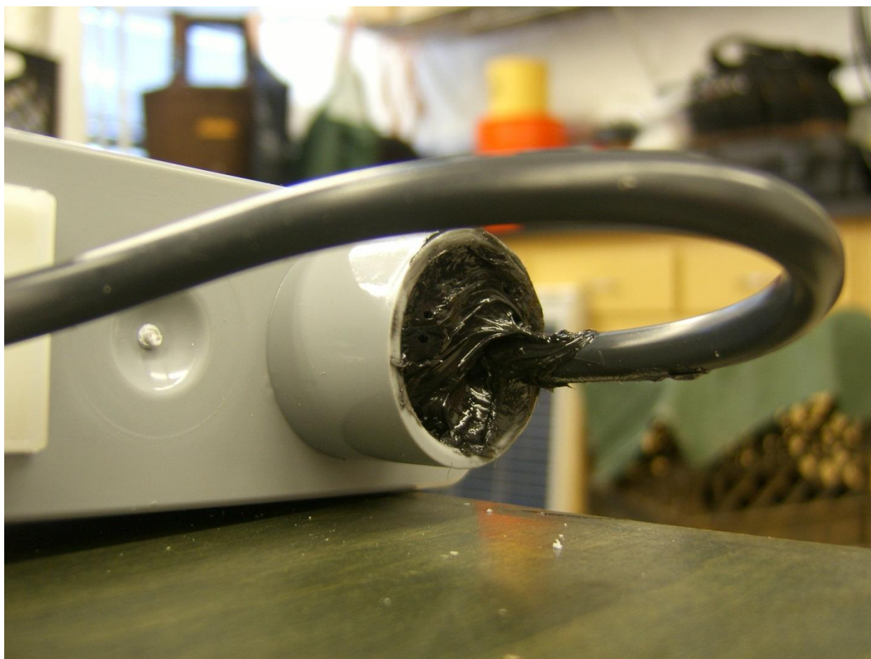
Figure S14 – The first coat of silicone sealant, applied from the outside of the box.
