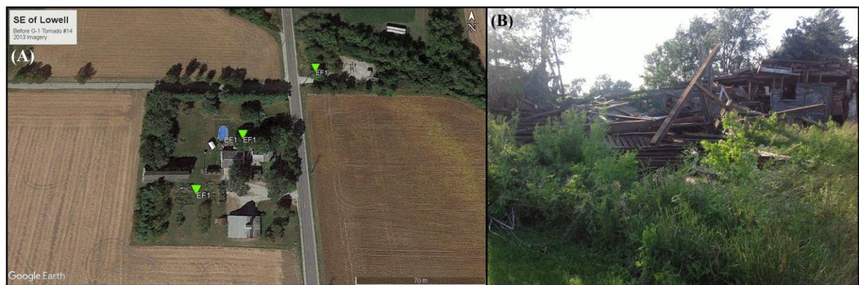
Figure A9: a) Before-and-after loop of Google Earth satellite imagery showing damage to a farmstead caused by tornado 14 of mesovortex G-1. b) Destroyed barn at the farmstead shown in (a), as found on the first ground survey. Click image to enlarge and animate.
