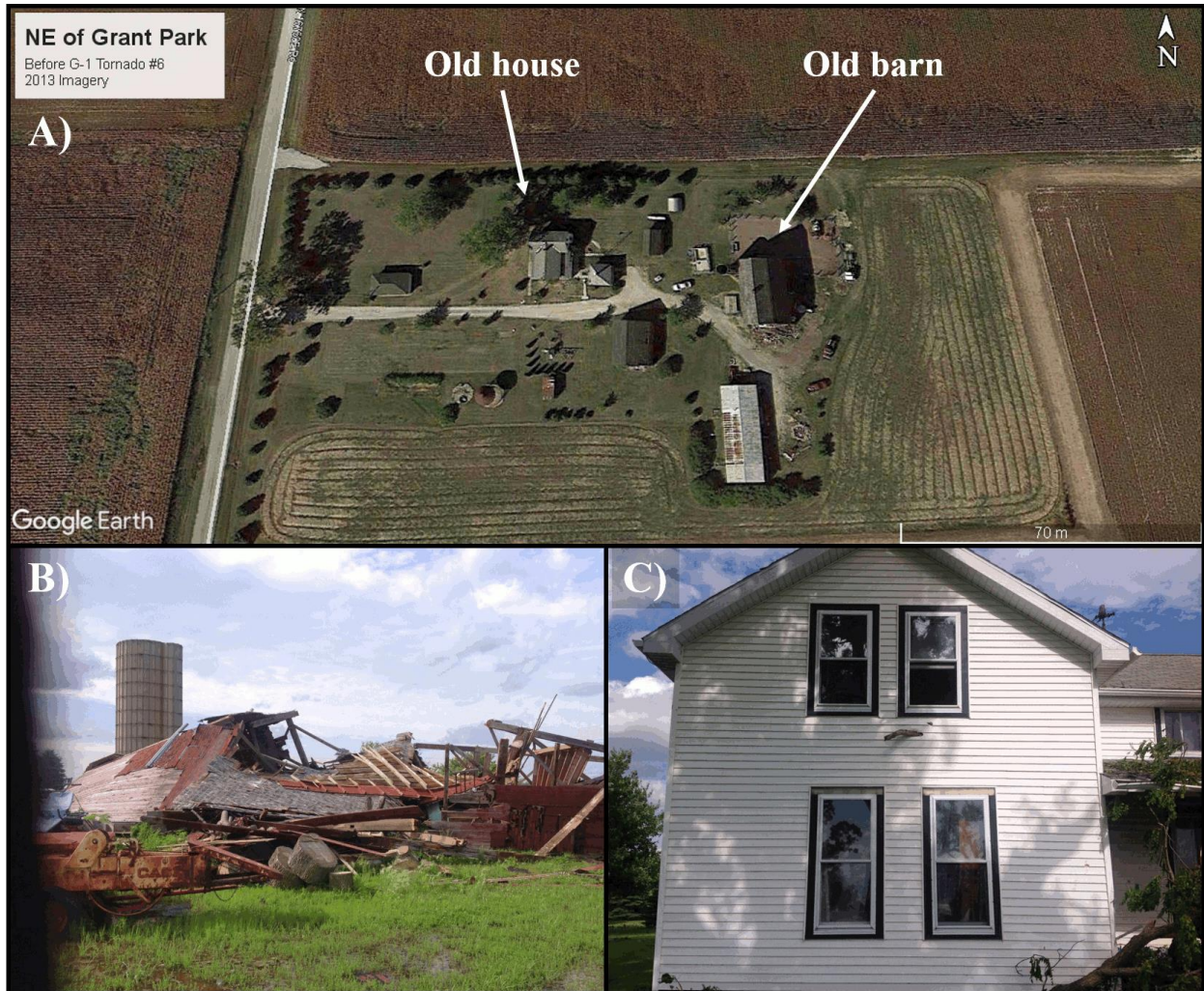
Figure A2: a) Before-and-after Google Earth satellite loop of the farmstead most heavily impacted by tornado 6 of mesovortex G-1. b) Picture of the destroyed three-story barn. c) A tree limb impaled into a second-story bedroom of the house on the farmstead. Click image to enlarge and animate.
