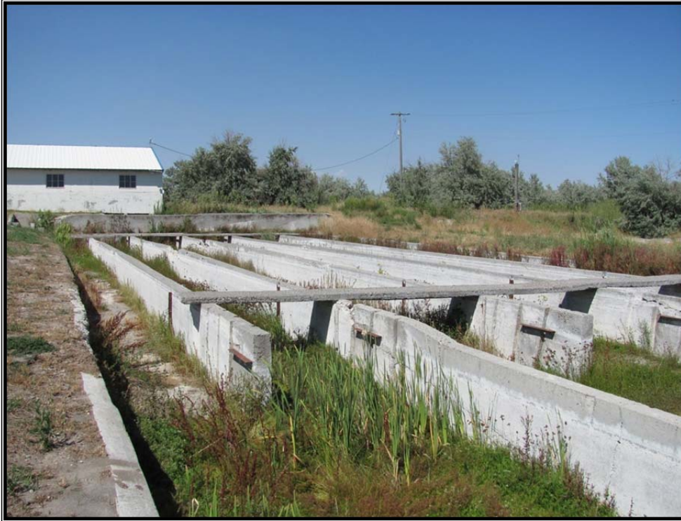
Figure 3.10-2: View of the Existing Raceways to the North
