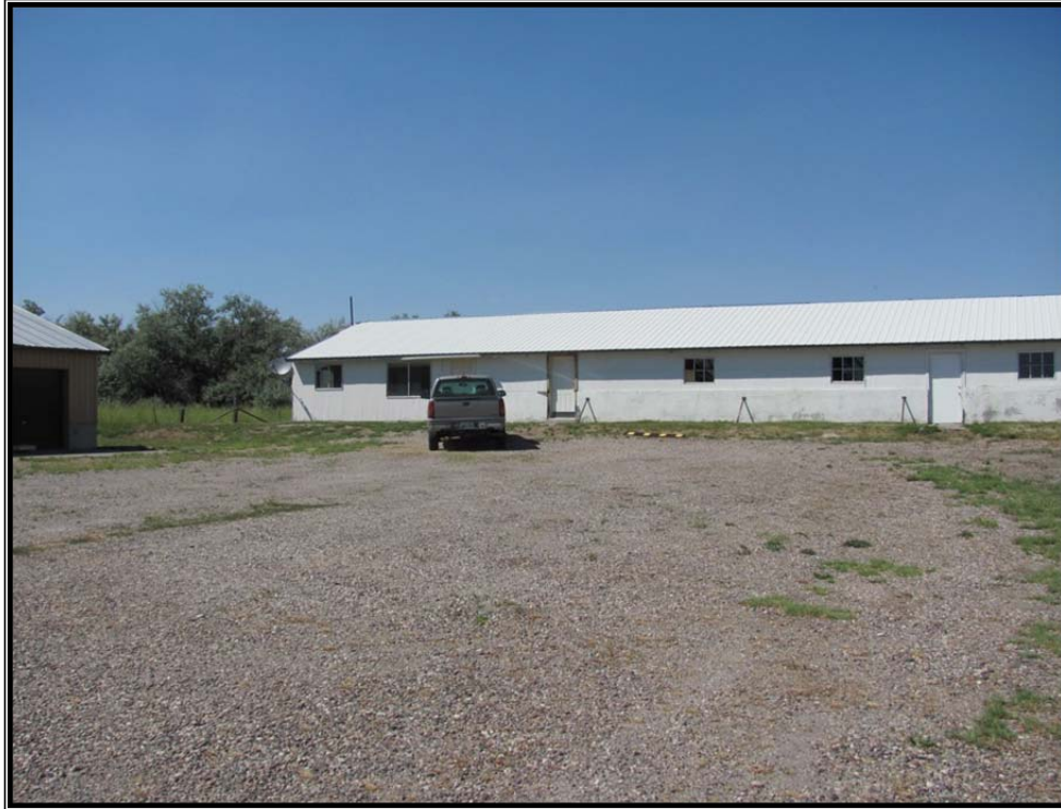
Figure 3.10-1. View of the Existing Hatchery Building to the North
