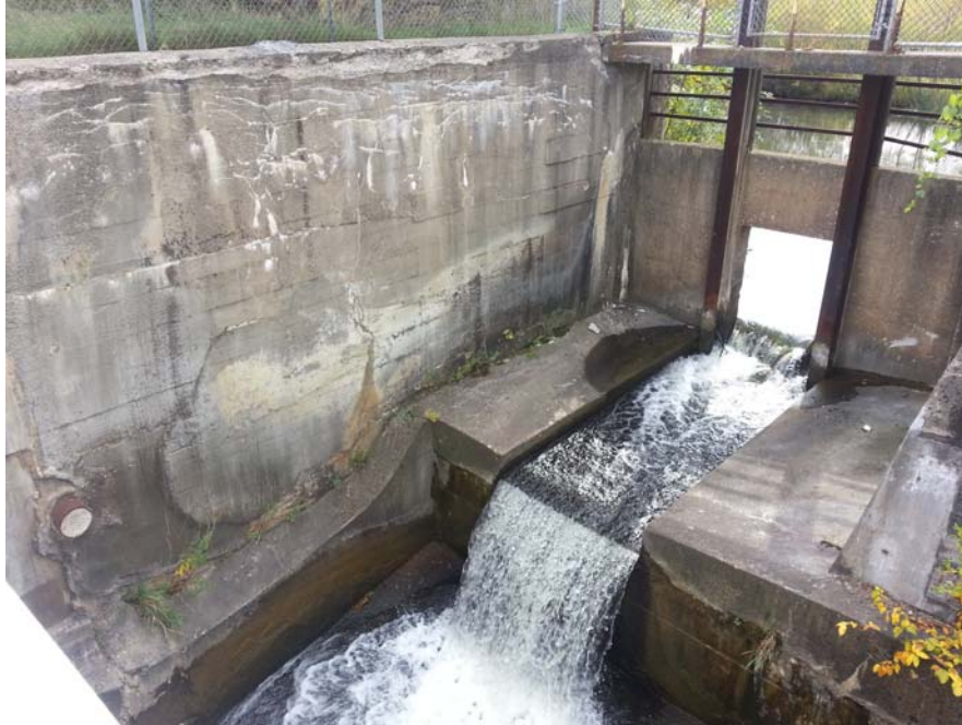
Figure 4. Alcott Street dam structure.
