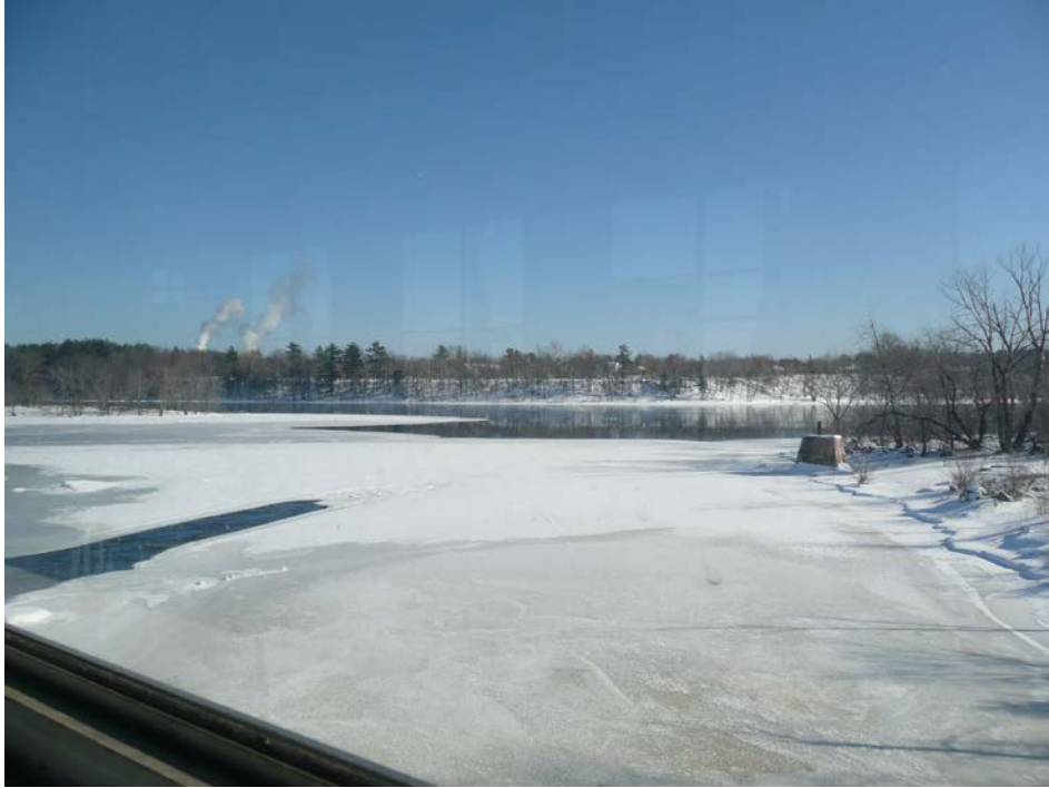
Figure 10. View of confluence of Piscataquis and Penobscot Rivers (downstream) from the Howland powerhouse on the southern bank of the Piscataquis River. (Source: Staff)
