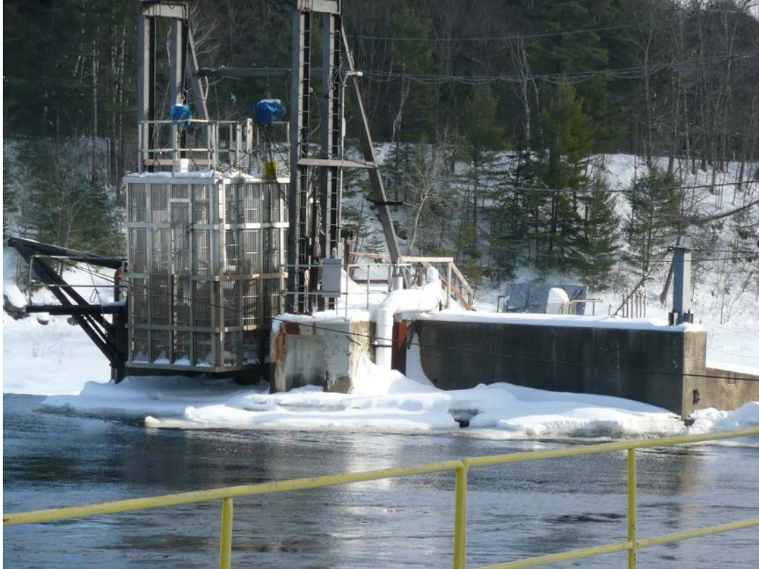
Figure 7. View of Veazie fish lift and trapping facility accessed by cableway from west bank of the Penobscot River. (Source: Staff)
