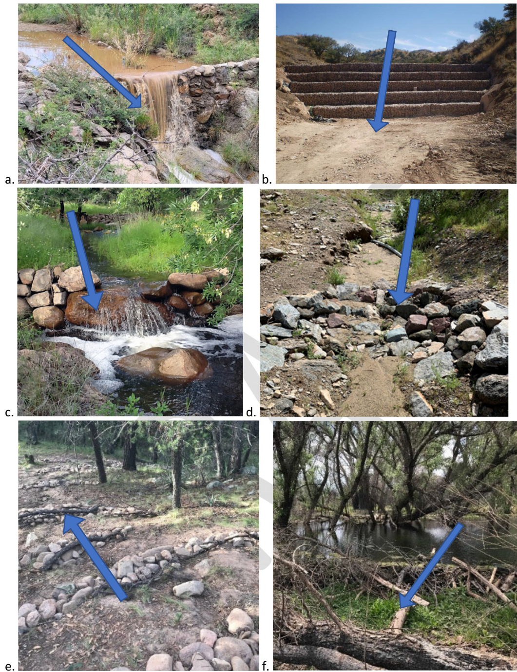
Fig. 2. Examples of human- and beaver-made NIDS, including a) leaky weirs (photo by Josiah Austin), b.) gabion (Photo by Andrea Prichard (Norman et al., 2010b)), c.) check dams (photo by Jeremiah Liebowitz), d) one-rock dams (Photo by Deborah Tosline (Tosline et al., 2020)); e.) trincheras (Photo by Valer Clark), and f.) a beaver dam, where blue arrows portray direction of flow.
