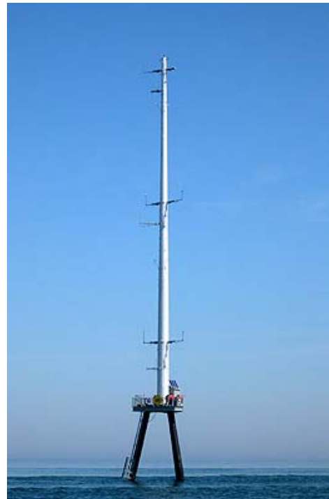
Figure 3-1. Cape Wind Meteorological Tower.
