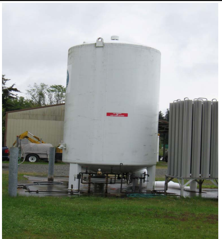
Photo 5: Ozone gas tank. All marine wastewater passes through the ozone treatment system before it is discharged to Clam Bay.
