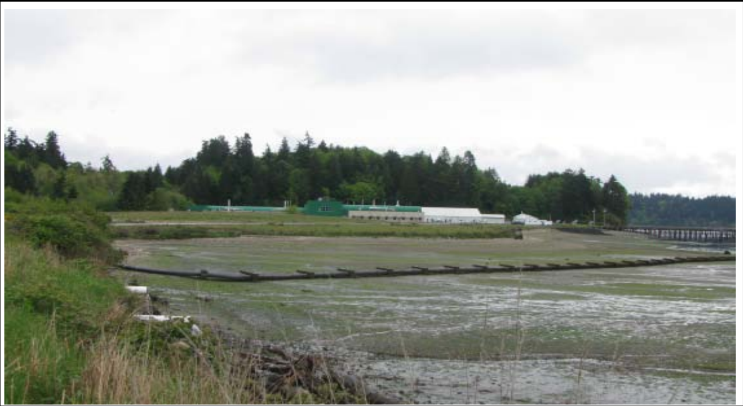
Photo 7: Clam Bay shoreline facing EPA Laboratory. Saltwater intake pipe, center.
