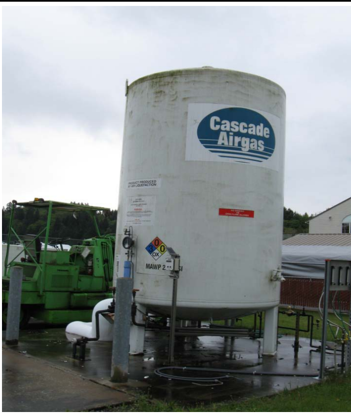
Photo 5: Ozone gas tank. All marine wastewater passes through the ozone treatment system before it is discharged to Clam Bay.
