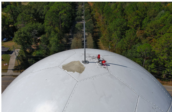
Image 12: Inspection of a NEXRAD radome via UAS. Photo: NOAA
