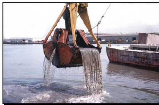
Figure 8. Mechanical dredge (clamshell bucket and barge).
