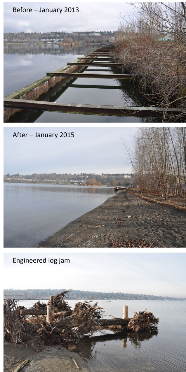
Figure 2. Photos of the Shuffleton Flume site. The top 2 photos display before and after the flume structure was removed (photos were taken at the same approximate location). The bottom photo is of one of the engineered log jams (ELJ; photo was taken on 15 Jan 2015, shortly after construction). From January to June, the lake level rises approximately 0.6 m to inundate much of the ELJ shown.
